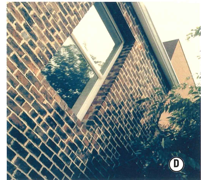
RAW MASONRY JAMBS EXPOSED
