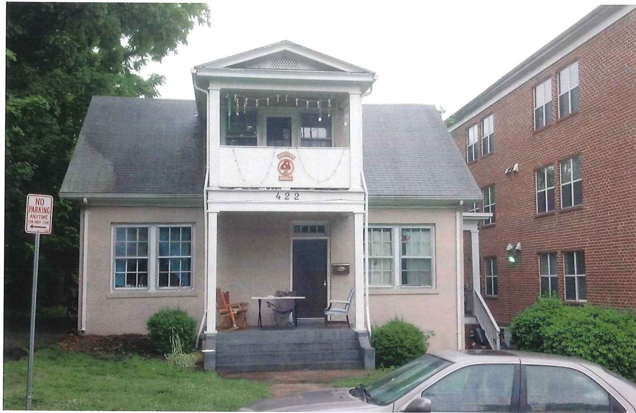
422 17th St N.W. - Stucco rooming house to remain
