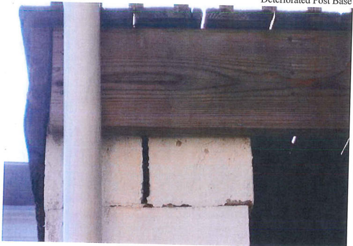
Rear Porch Pier
