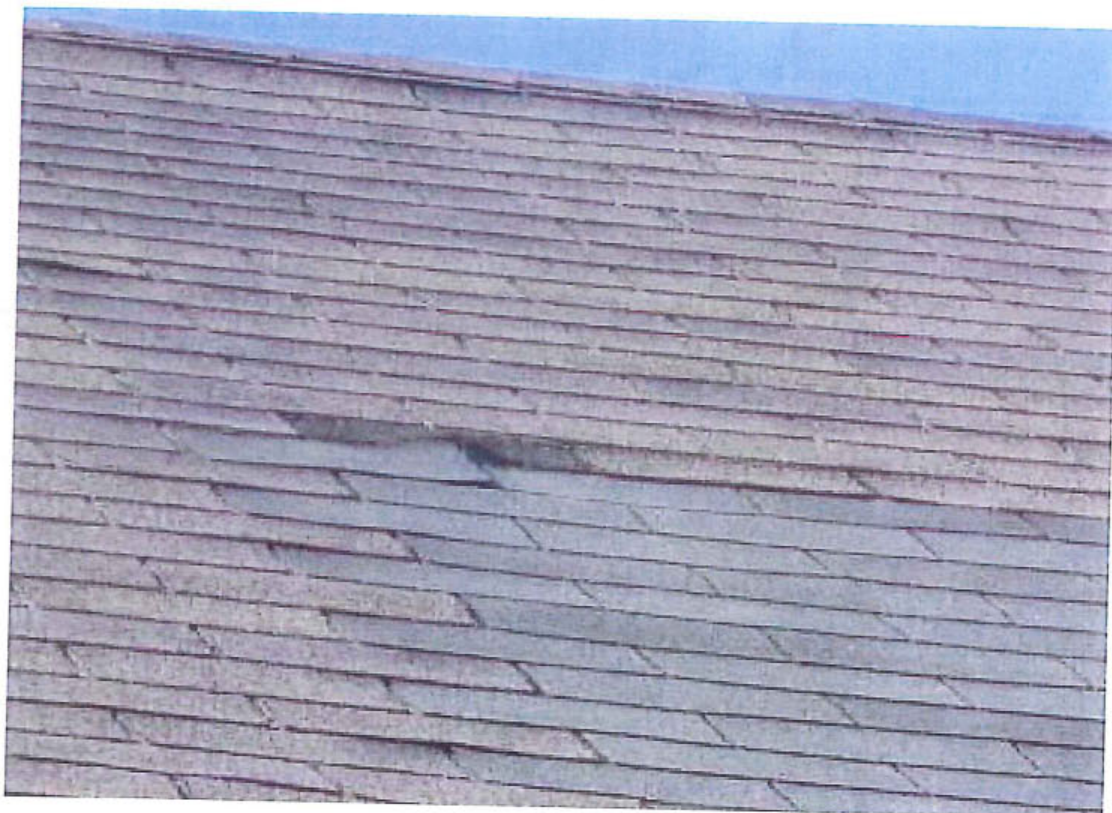
Roof Shingles / Patch
