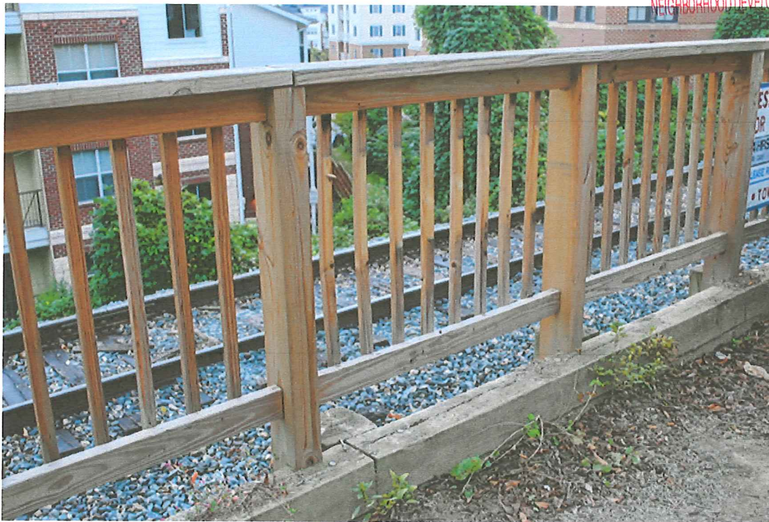
Existing rail across Elliewood Ave from property. Rail for deck and walk to be similarly constructed and stained grey.
