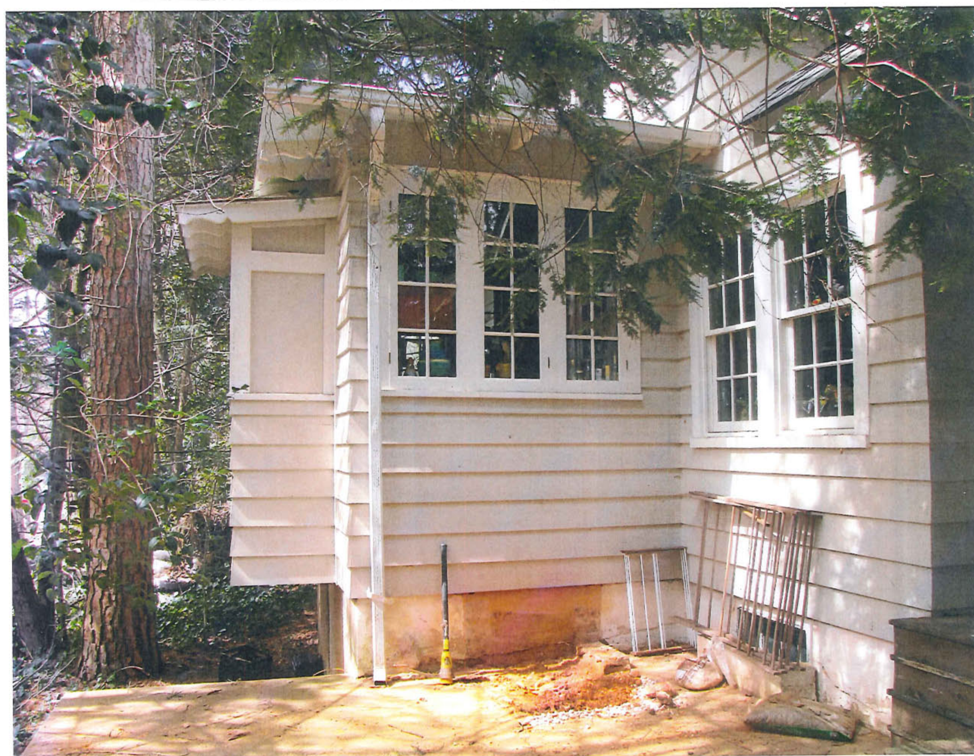
PATIO & ORIGINAL HOUSE
