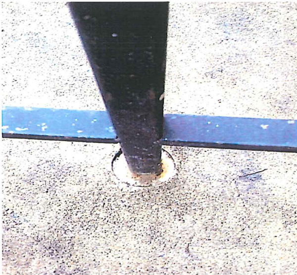
Epoxy for Middle Support
