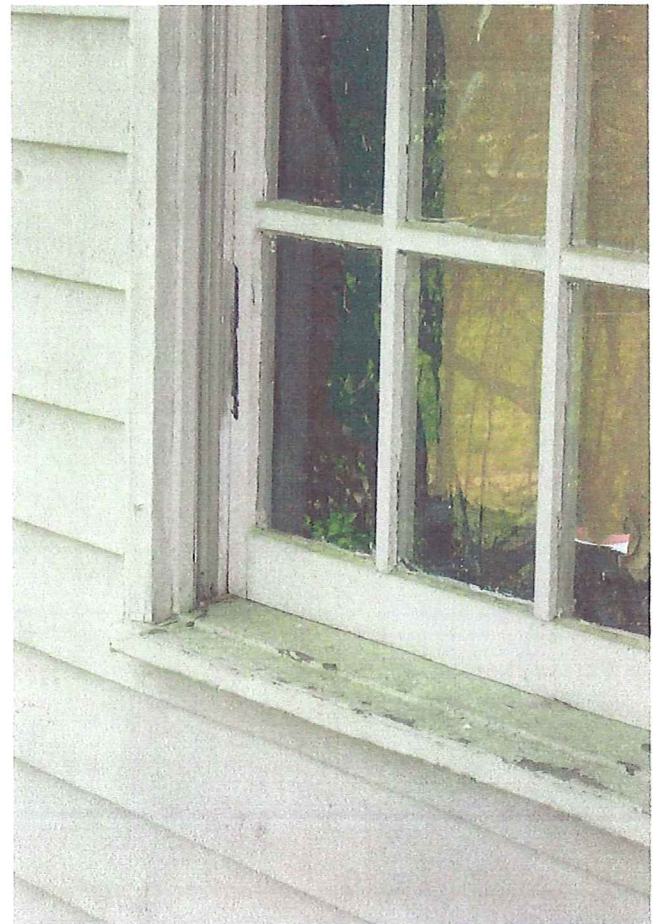
SOUTH "PORCH" WINDOW |
