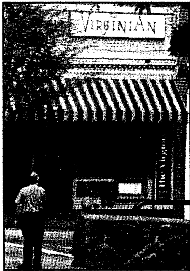
Progress photo by Matt Gentry
