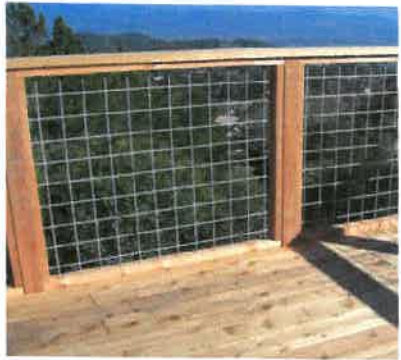
Ex. Wire mesh infill panels
