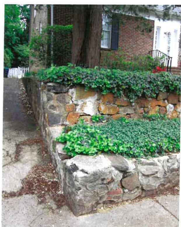
Stone retaining wall at chamaecyparis
