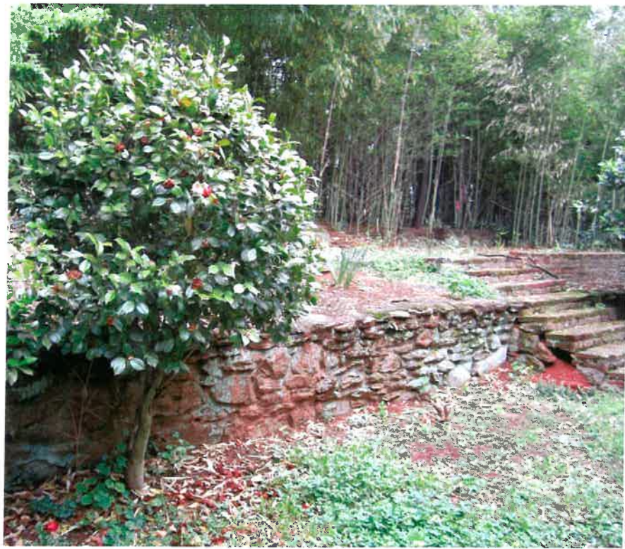
Rear yard wall, steps, and terrace
