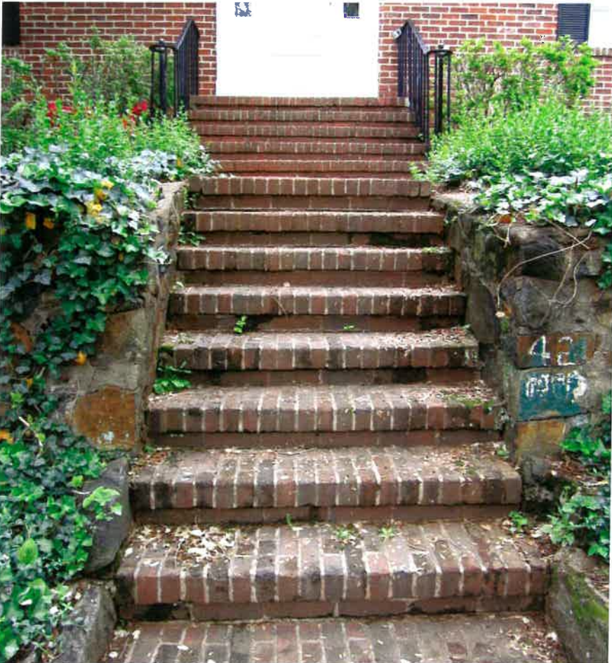
Front yard steps and walls
