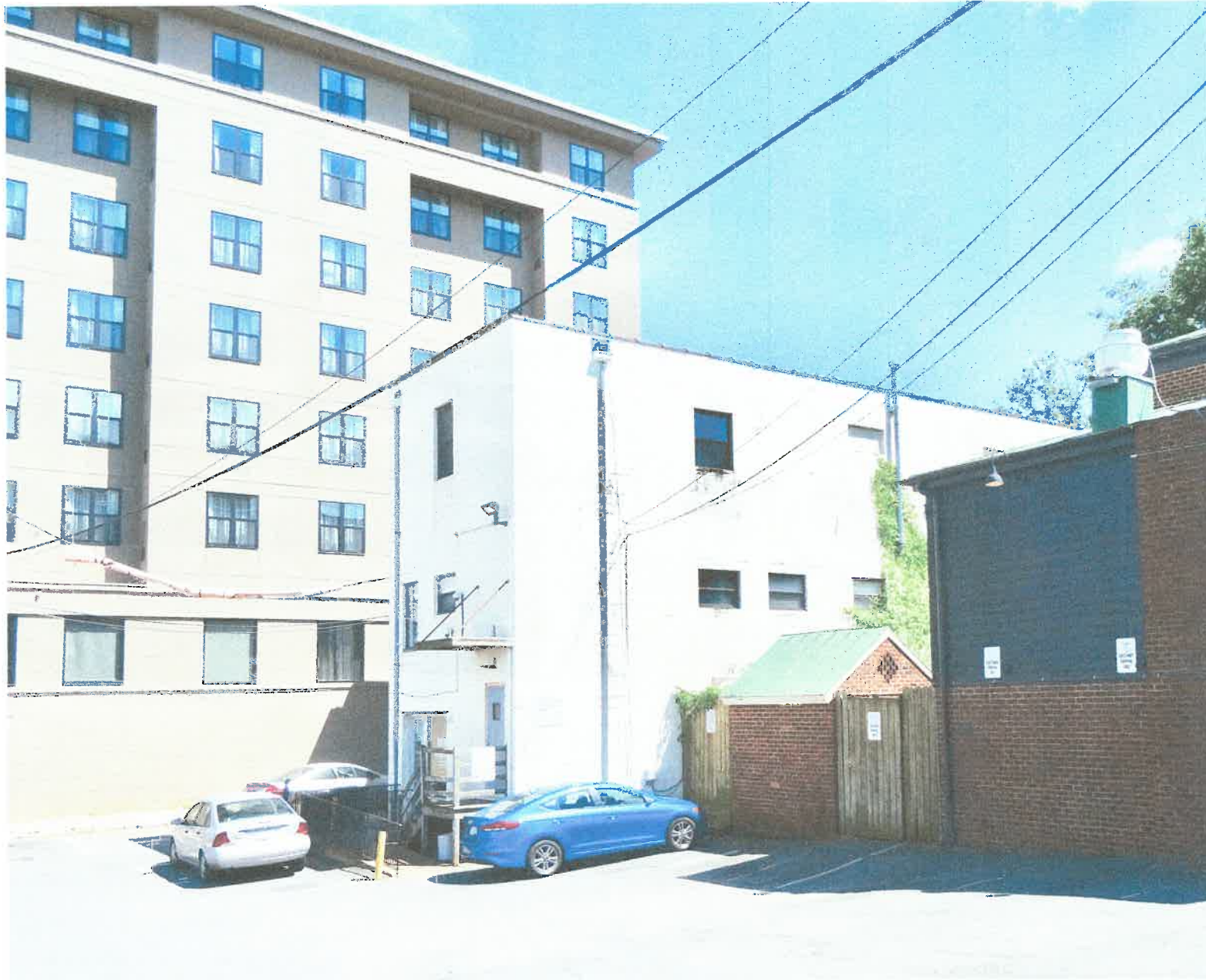
VIEW ON 4TH STREET NW FROM EAST SIDEWALK LOOKING SOUTHEAST
