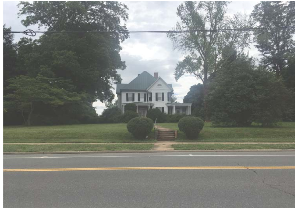
VIEW OF 834 LOCUST AVE FROM ACROSS STREET
