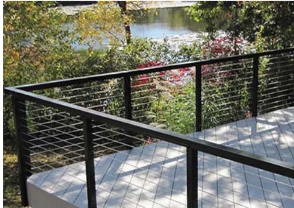
CABLE RAIL WITH STEEL POSTS
