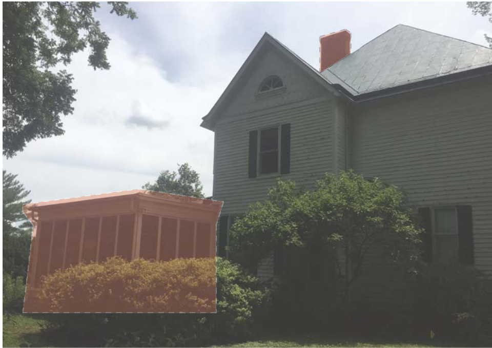
THREE SEASONS ROOM TO BE REMOVED
