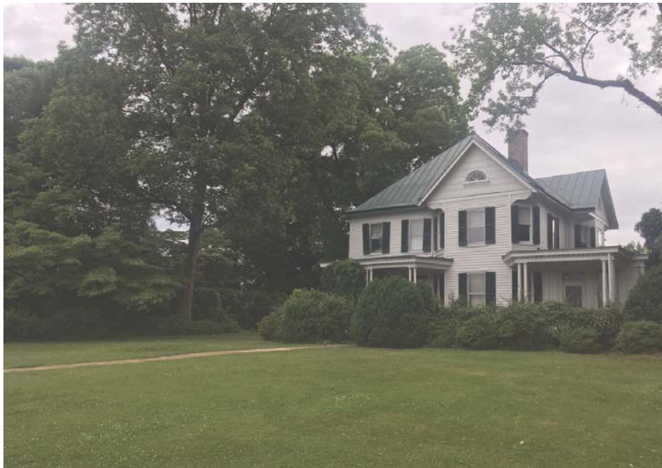
NO VISIBILITY OF ADJACENT HOME ON LEFT
