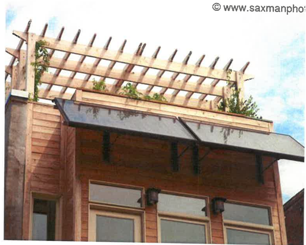
Building-integrated solar energy systems in residential districts
