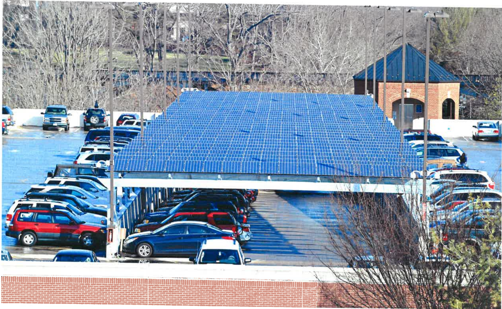
Parking Garage Canopies
