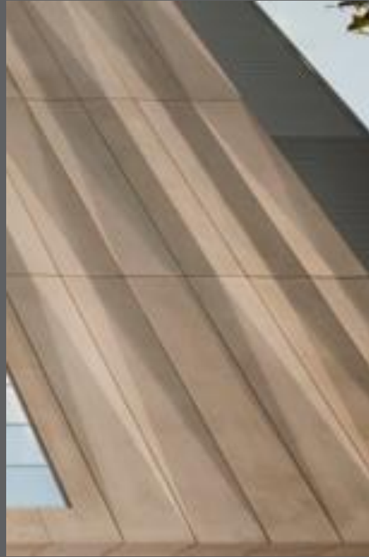
Intermittent Shadows Produced by Convex / Concave Faceted Panels
