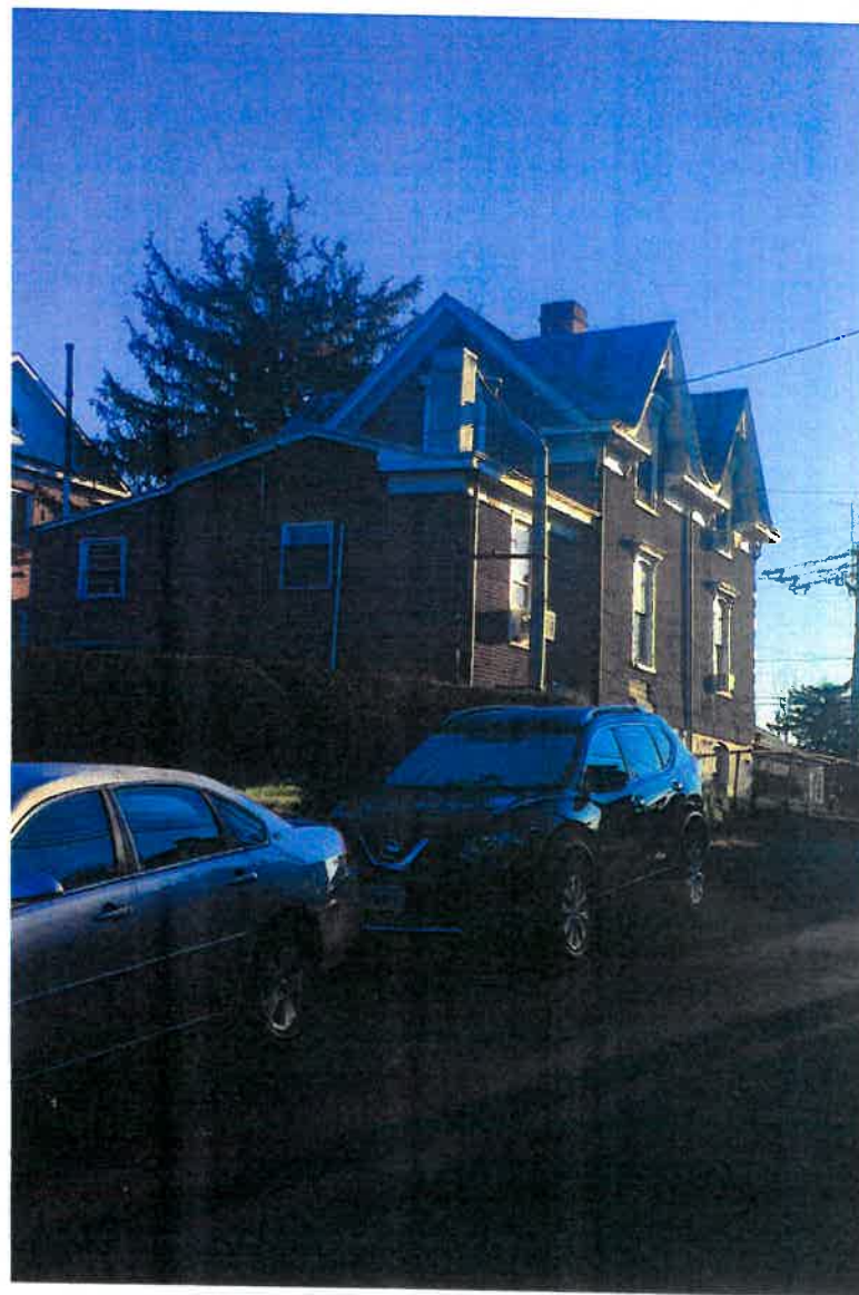
OAK STREET FACADE
