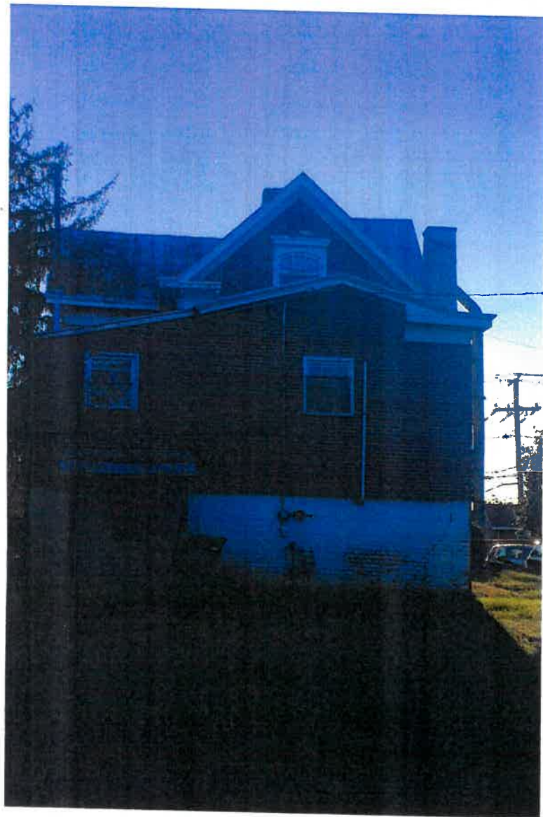
REAR FACADE 413 RIDGE STREET
