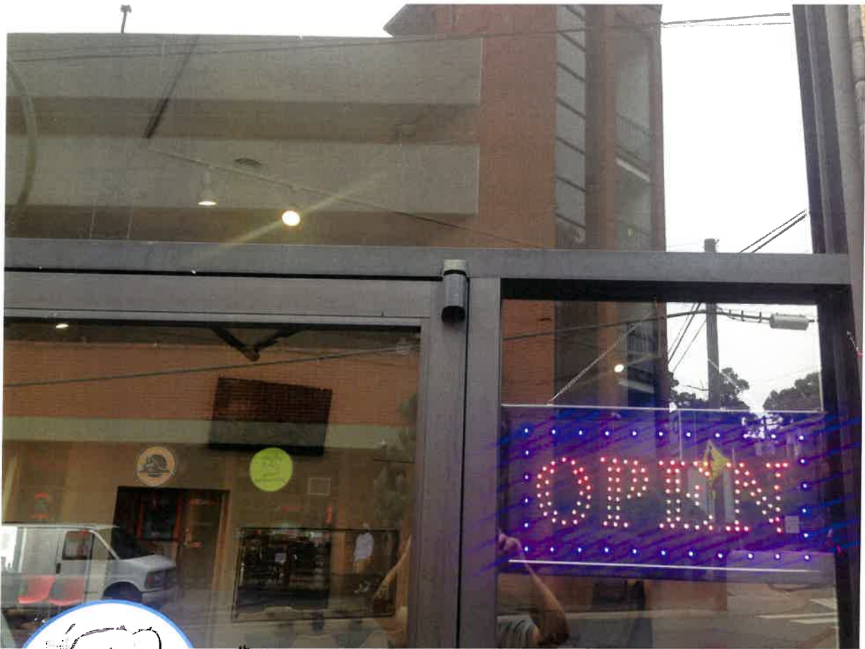
Existing storefront on 14 th Street NW. Proposed window and door to match color and material.
