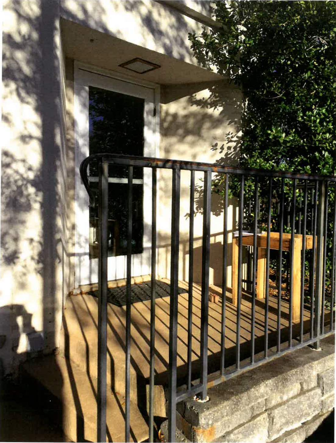
VIEW OF STAIR TOWER ENTRANCE
