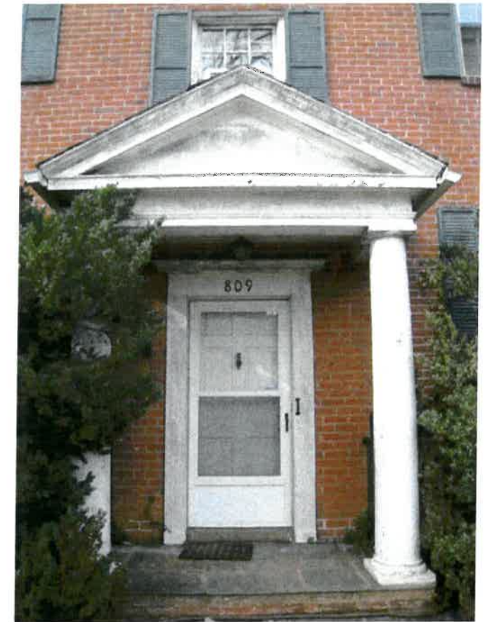
FRONT PORCH DETAIL
