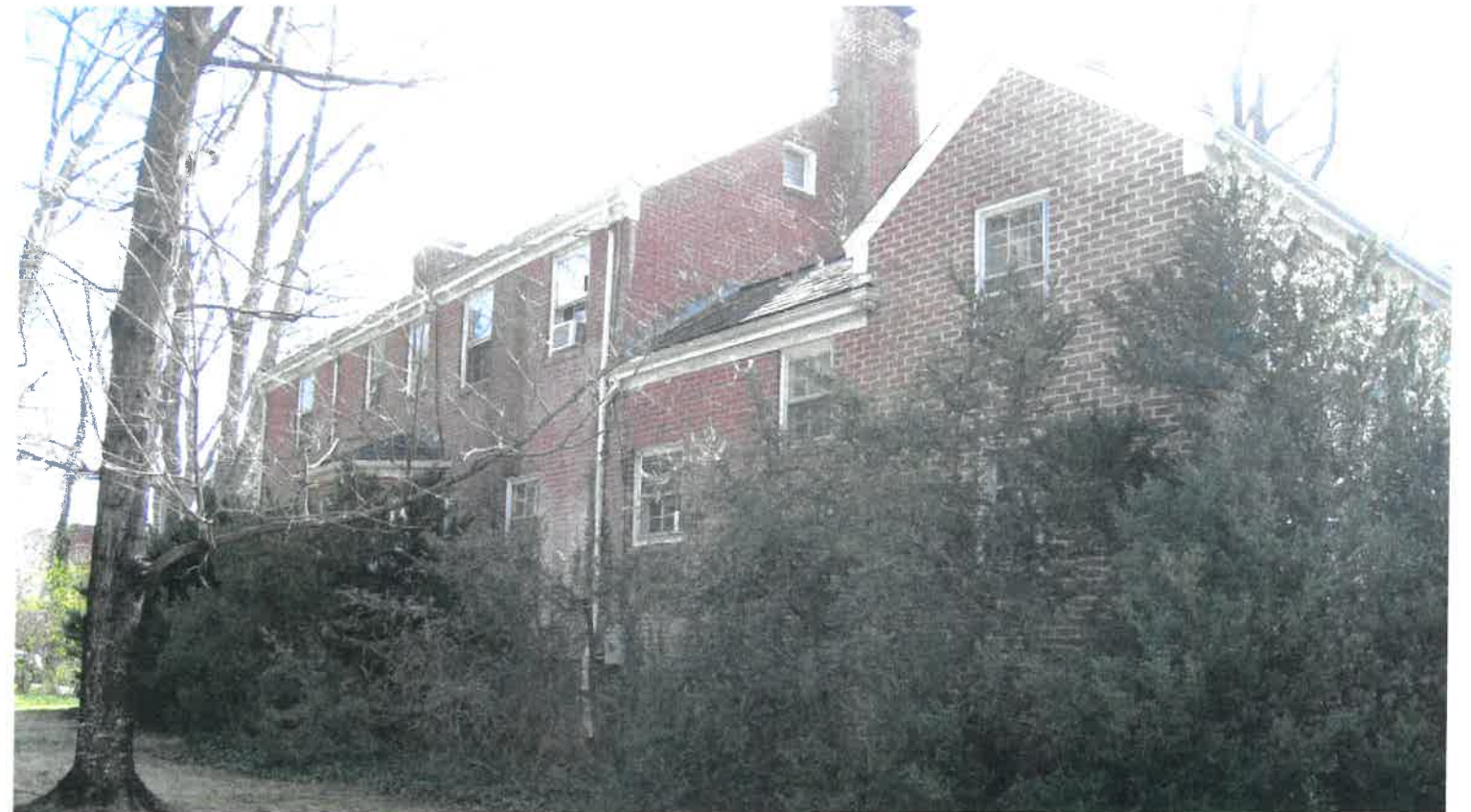
REAR YARD ELEVATION FROM WEST
