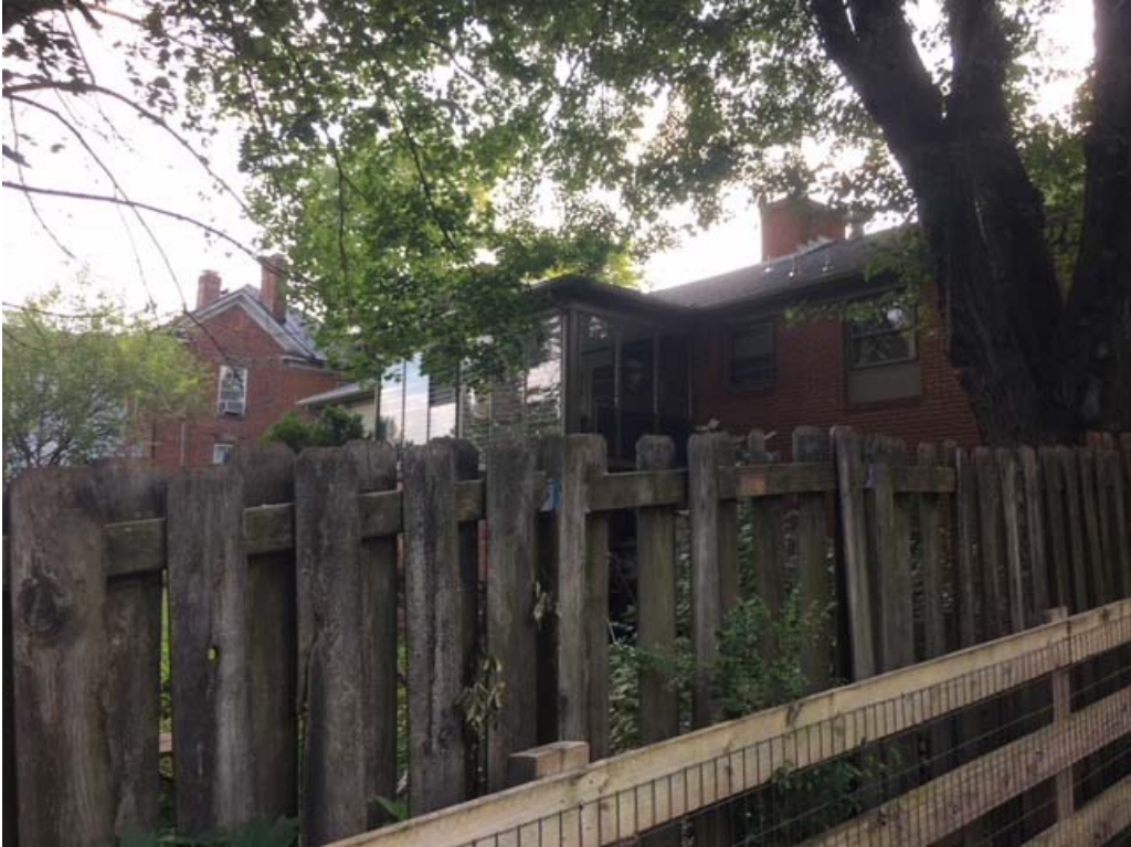
Adjacent rear porch
