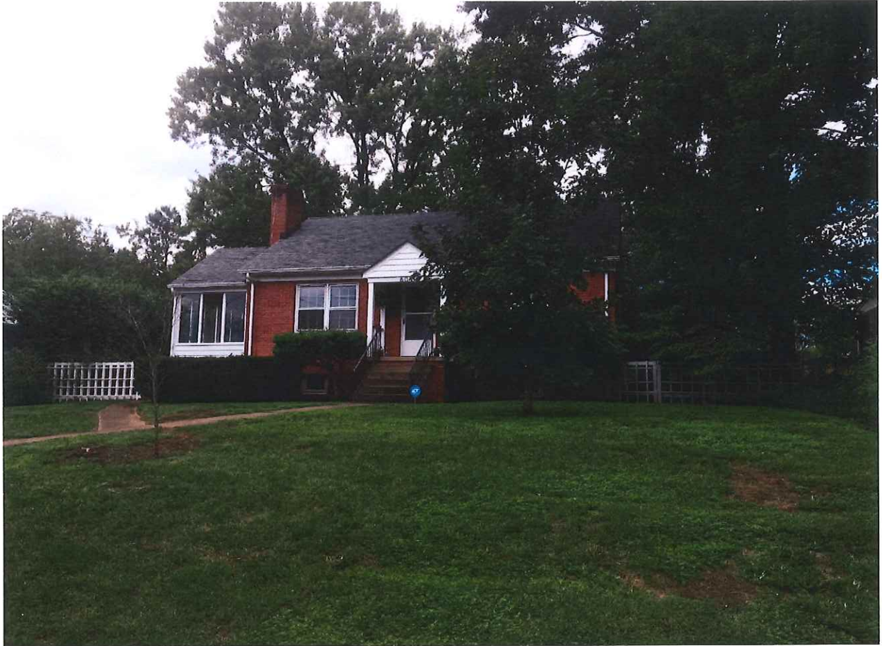
Front of House—more on right side of house
