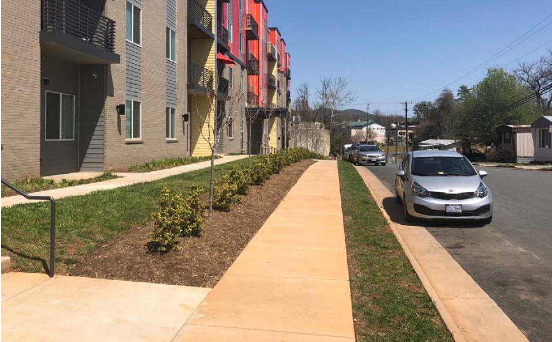
Picture of Carlton Avenue Streetscape
