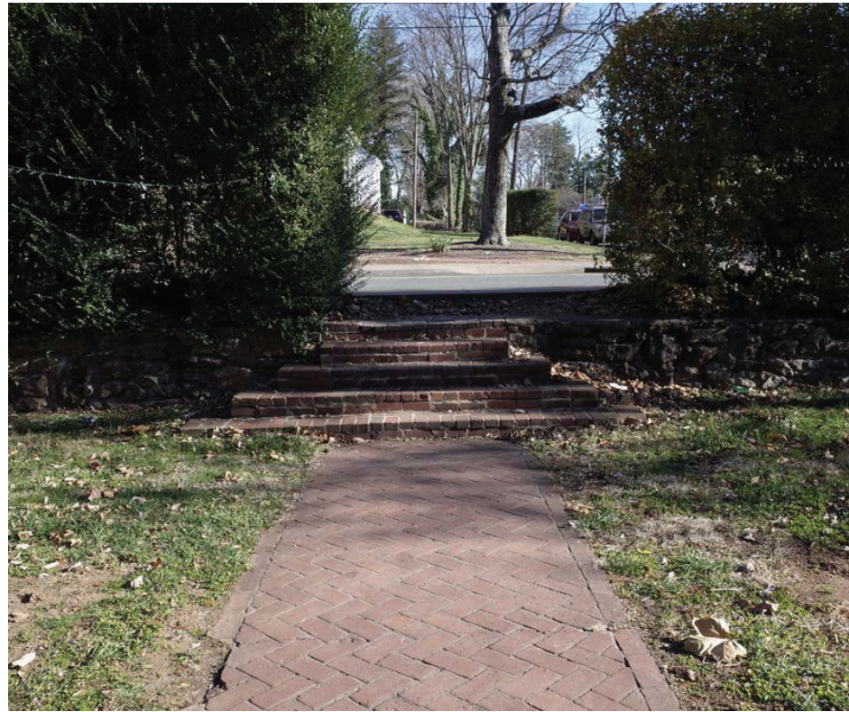
EVERGREEN HEDGE, ENTRY STAIR, AND SITE WALL IMAGE TAKEN FROM ADJACENT PROPERTY (513 RUGBY ROAD)
