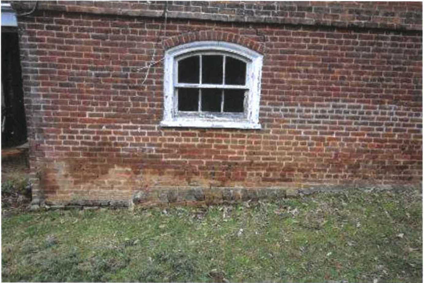
Portland Cement repointing
