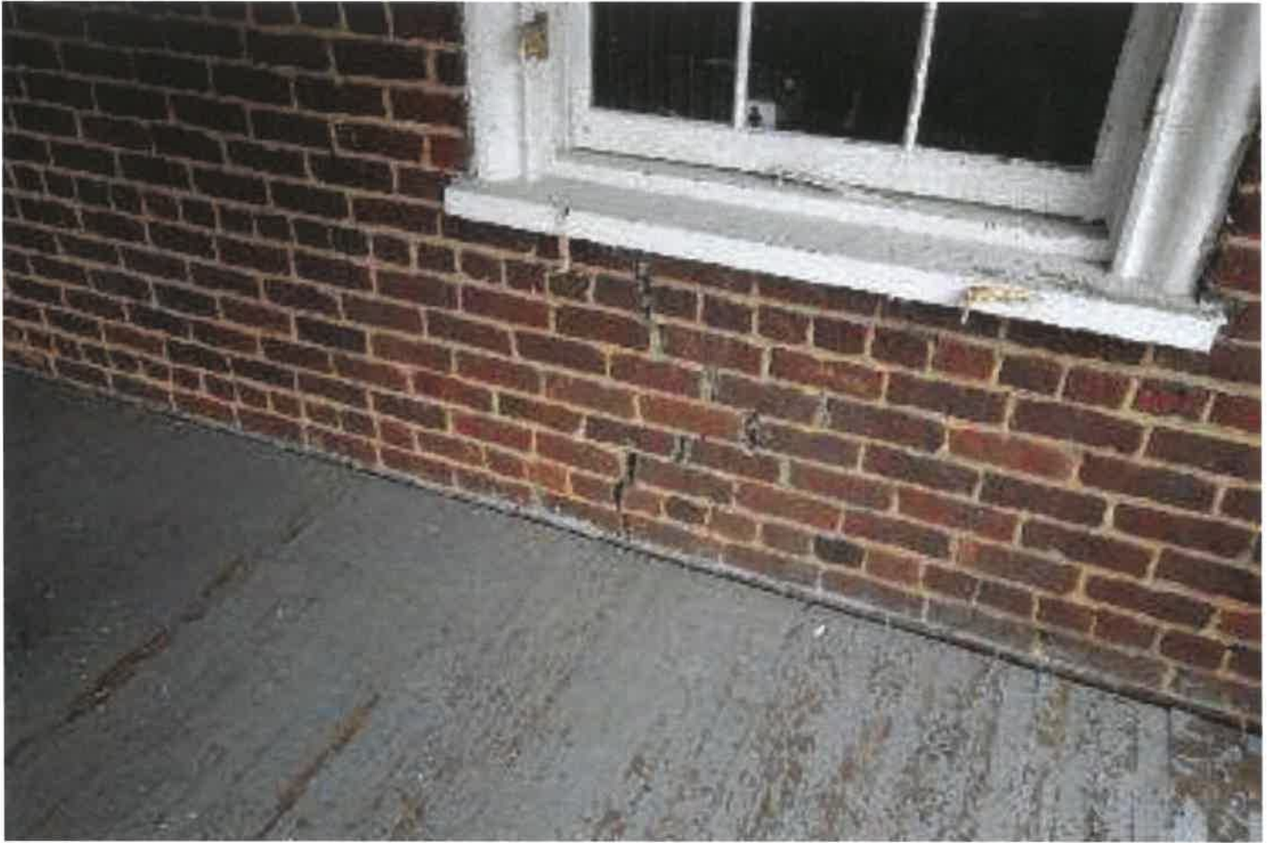
Masonry cracks
