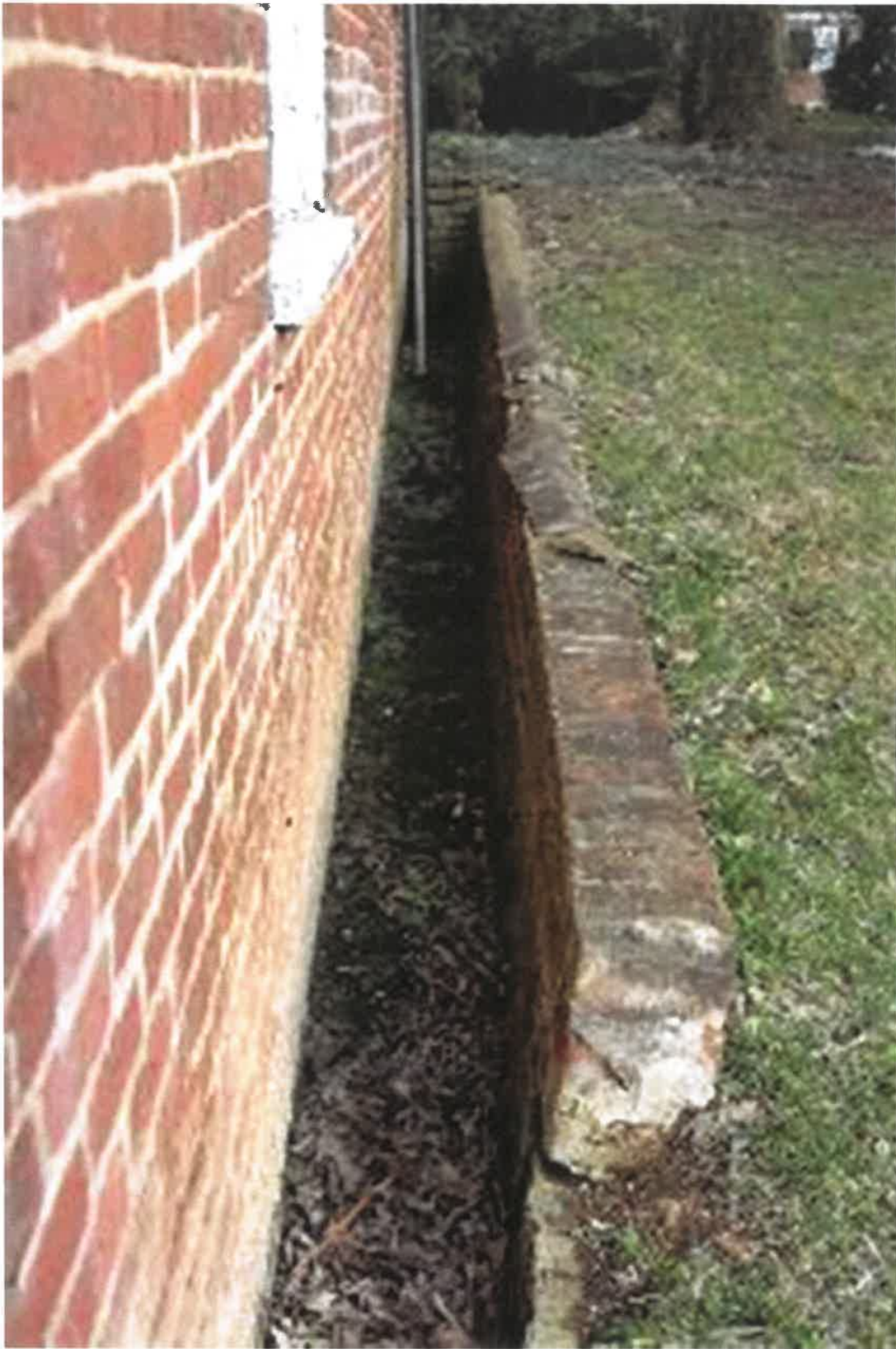
Perimeter Brick 'Moat'
