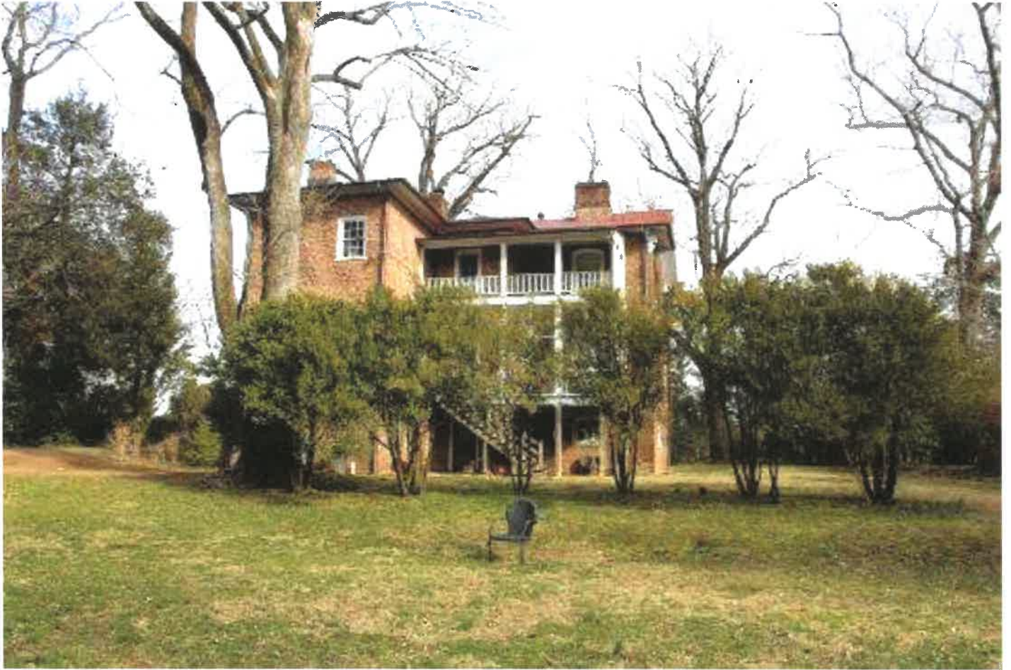
West Elevation (1920s Wing on the Left, 1861 Original House on the Right behind 1920s Porch)
