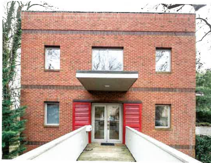
West (front facing First St.)
