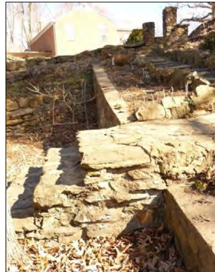
Photo 12: Details of Multi-Stone Treaded Stairs Leading West into Central Terrace (Dovetail, February 2011).
