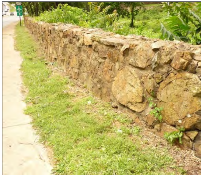
Photo 13: Details of Southwestern Junction Pre- and Post-Route 250 Bypass Stonework. Note different sizes in stone, mortar color, and coping (Dovetail, June 2011).
