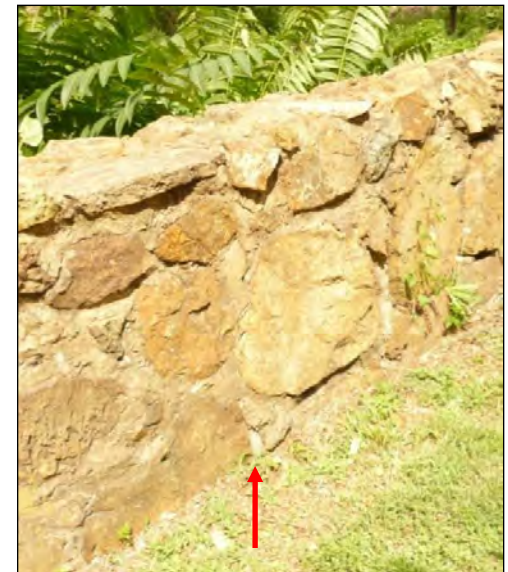
Photo 13: Details of Southwestern Junction Pre- and Post-Route 250 Bypass Stonework. Note different sizes in stone, mortar color, and coping (Dovetail, June 2011).
