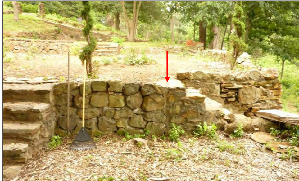
Photo 11: At Right, Detail of Central Terrace Walls and Stairs Looking East. Note “cold” joint where the multi-stone treaded stairs connect to older wall (Dovetail, June 2011).
