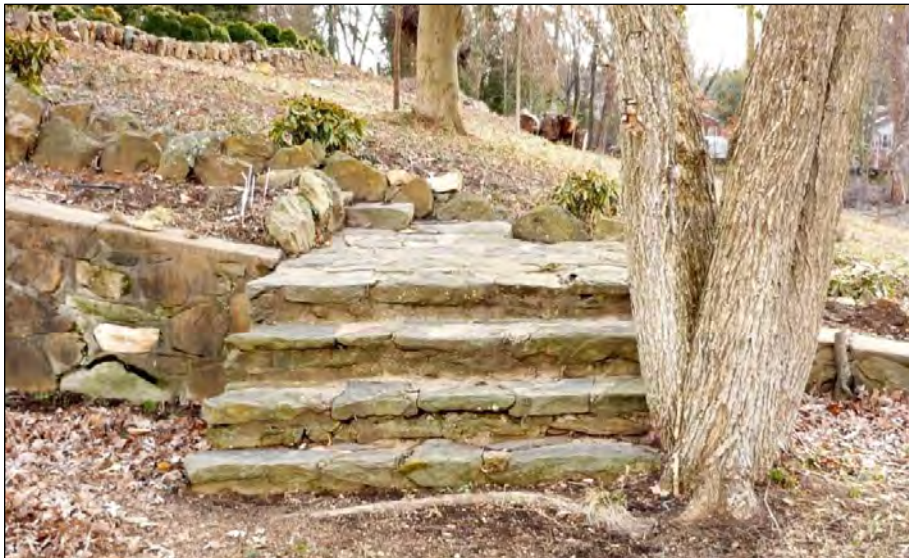
Photo 12: Details of Multi-Stone Treaded Stairs Leading West into Central Terrace (Dovetail, February 2011).
