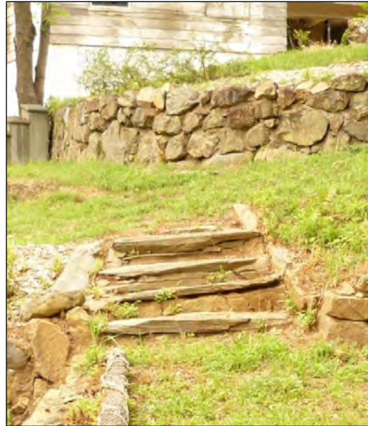
Photo 9: At Center and Right, Single-Stone Treaded Stairs in Formal Terraced Garden (Dovetail, June 2011 and February 2011).
