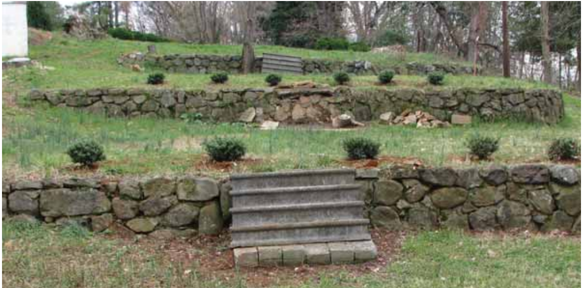
Upper terraces. Note missing stairs on central terrace. Building in upper left is an unused lunchroom likely associated with Rock Hill Academy (March 2011).
