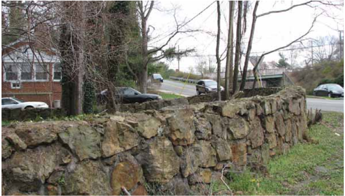
Perimeter stone wall (March 2011).
