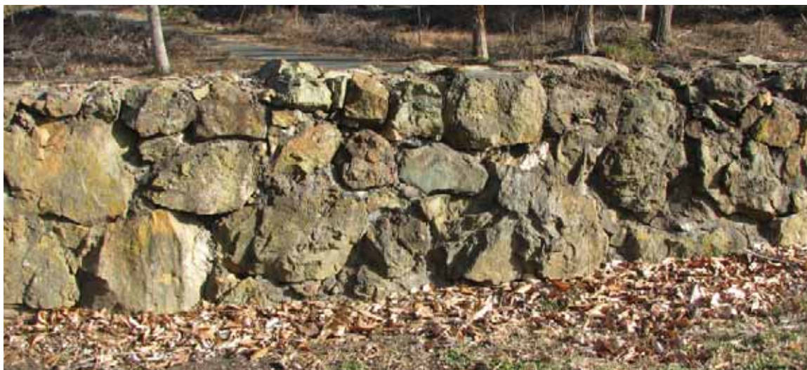
Southern boundary wall, near western gate post (February 2011).
