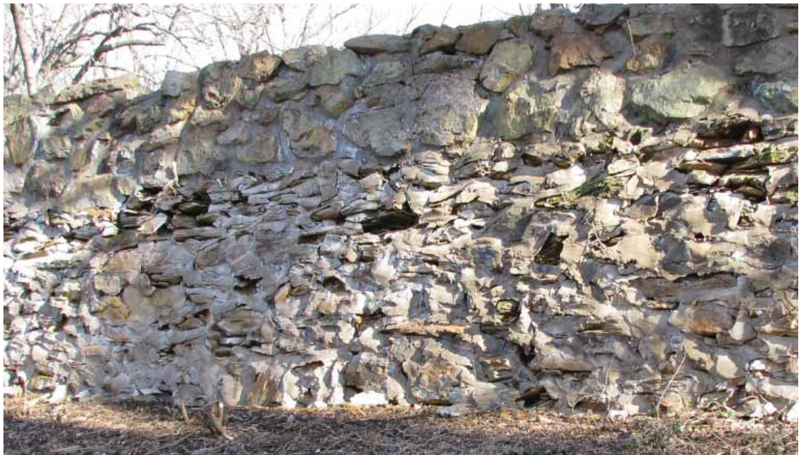
Contrasting stonework on terrace wall (February 2011).
