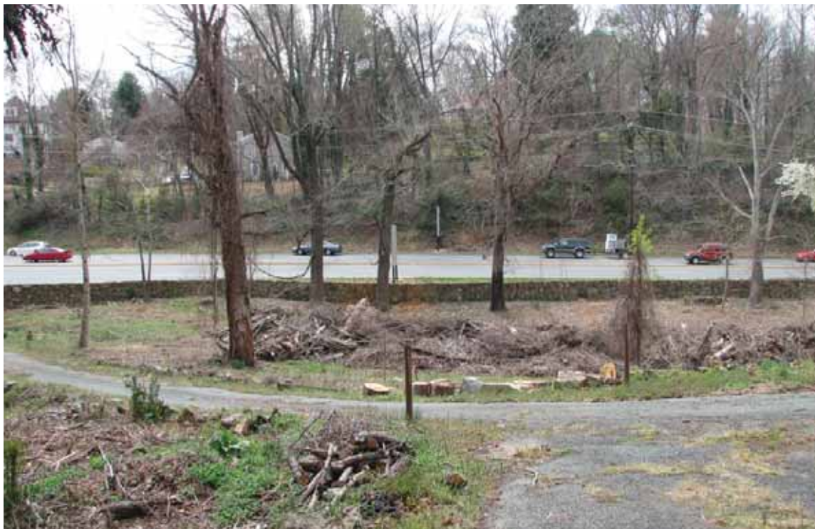
View to cleared area at the bottom of the slope, taken from the historic driveway. (March 2011).
