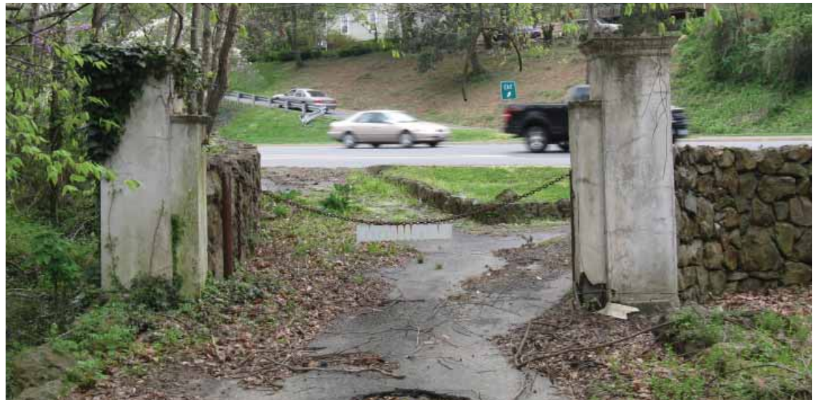
Entry gate columns (RKK).
