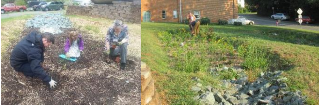
Sojourners Church Bioretention – funded through grants from the Rivanna Conservation Society and CCAP. LEFT: church volunteers plant the 2 bioretention cells with native plants. RIGHT: the practice in August 2015. Bioretention treats about 11,000 square feet of impervious cover.
