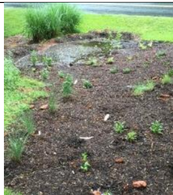
Rain Garden for residence
