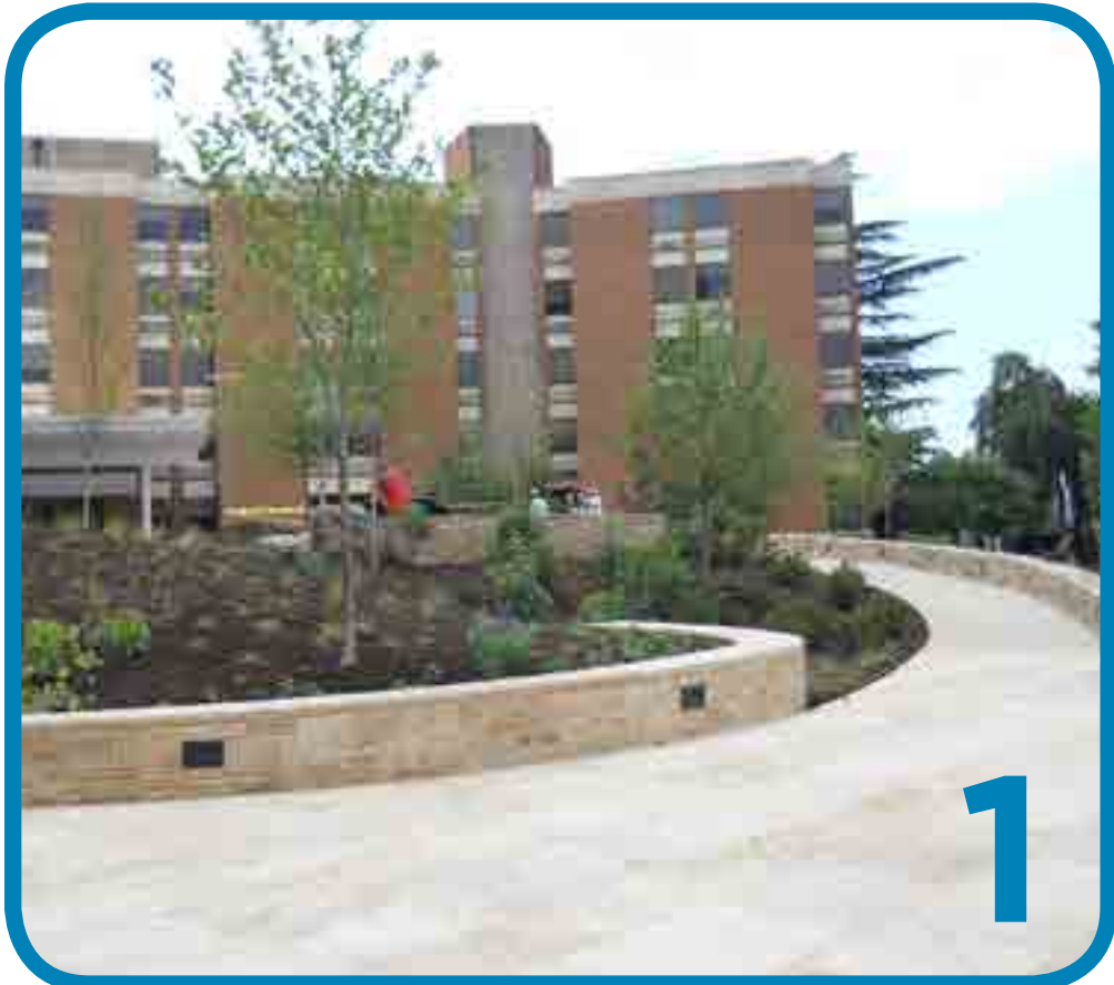
Jefferson Park Ave. Intersection
