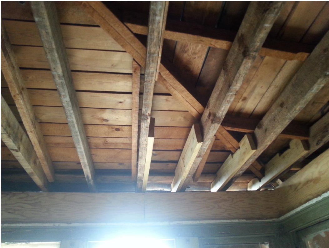
Photo 2 – Partially completed back roof repairs
