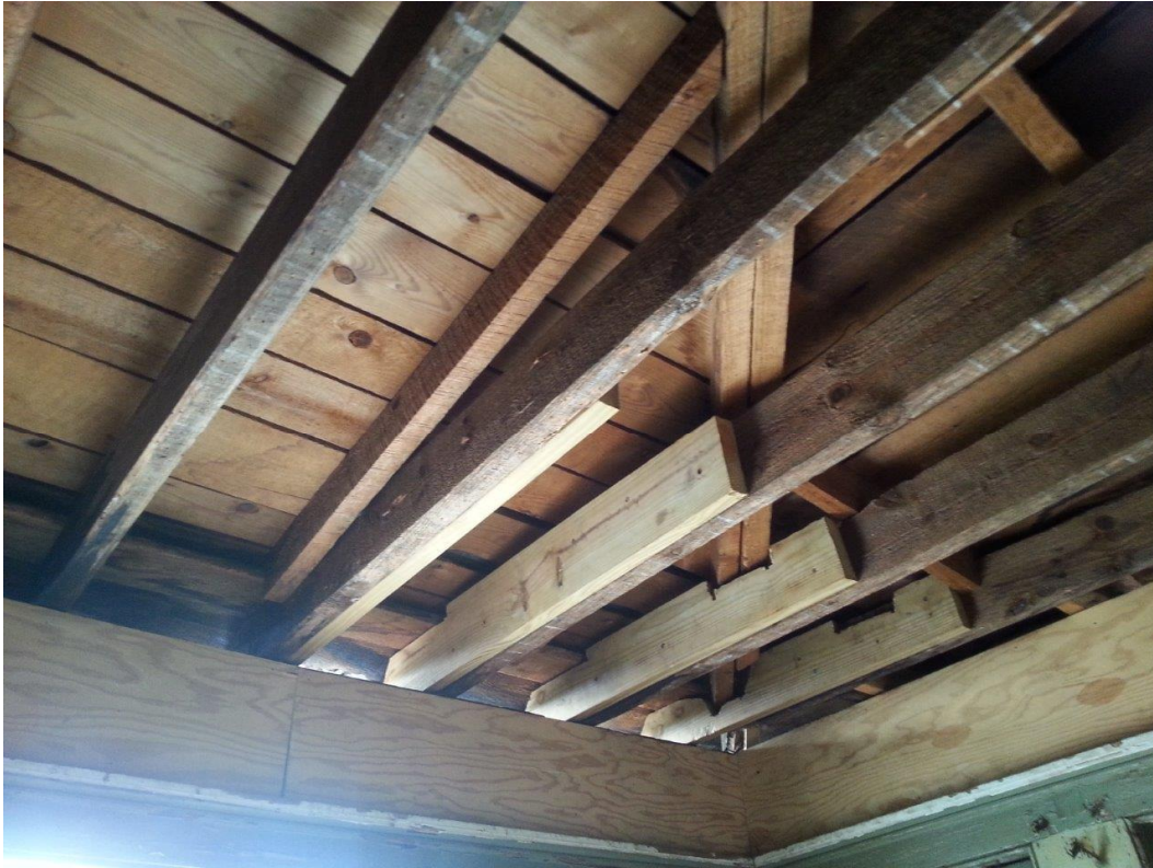
Photo 1 - Partially completed back roof repairs
