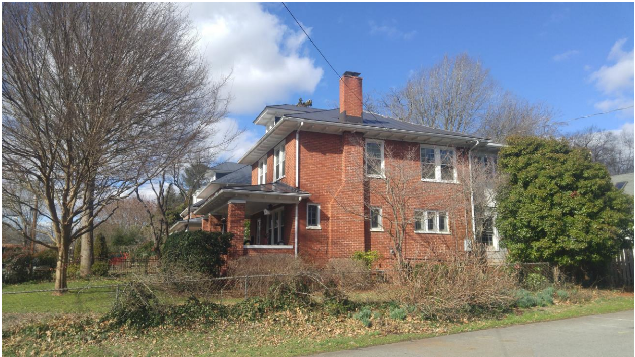
Figure 4: Oblique view, facing northwest, of subject building.
