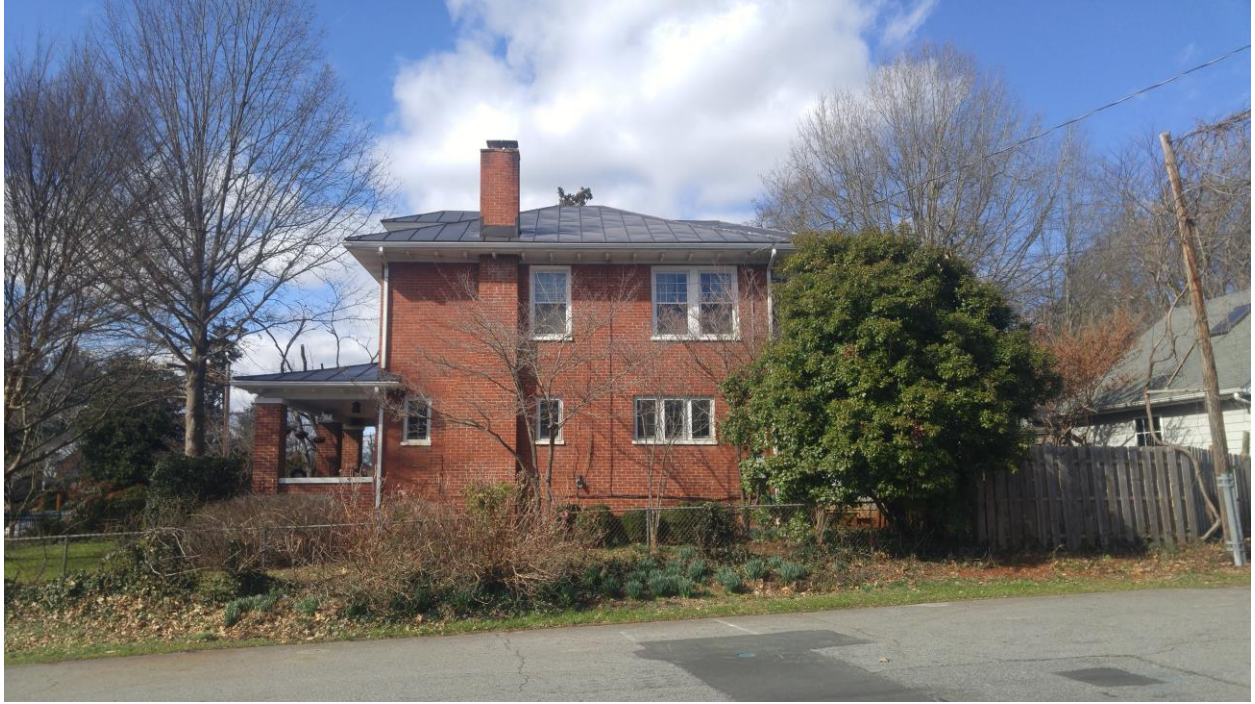
Figure 5: East elevation of subject building.
