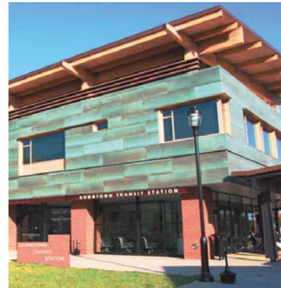
Figure 8 | CAT Downtown Transit Station
