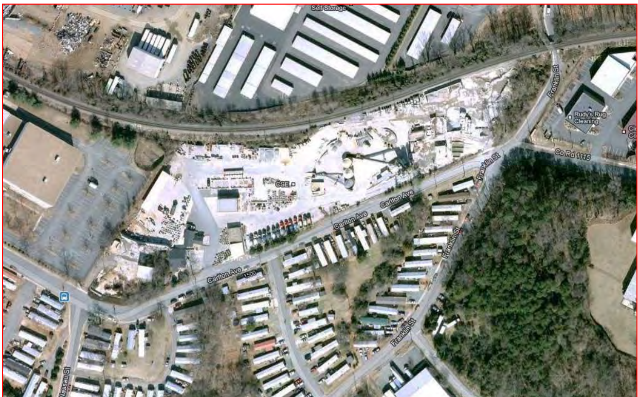
Figure 1: Existing Conditions – Allied Concrete Plant
