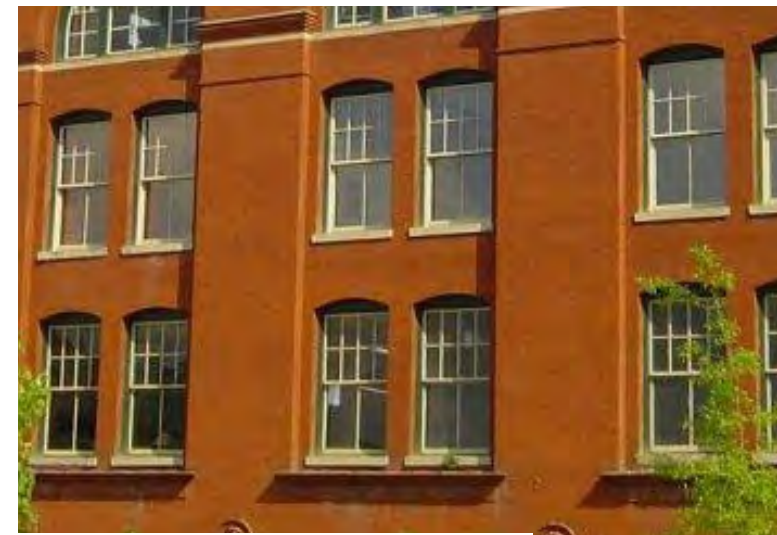
Aluminum Framed Fixed Windows in Brick
