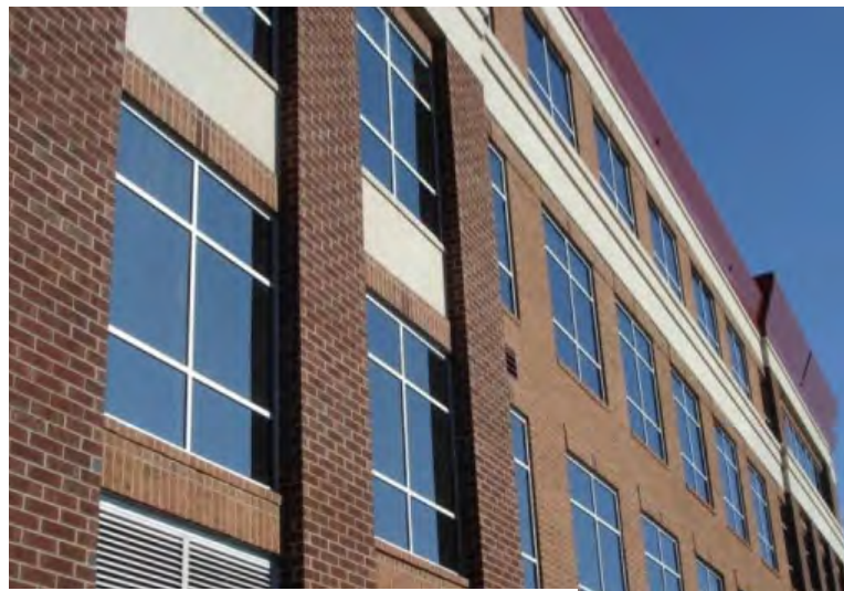
Aluminum Framed Fixed Windows in Brick
