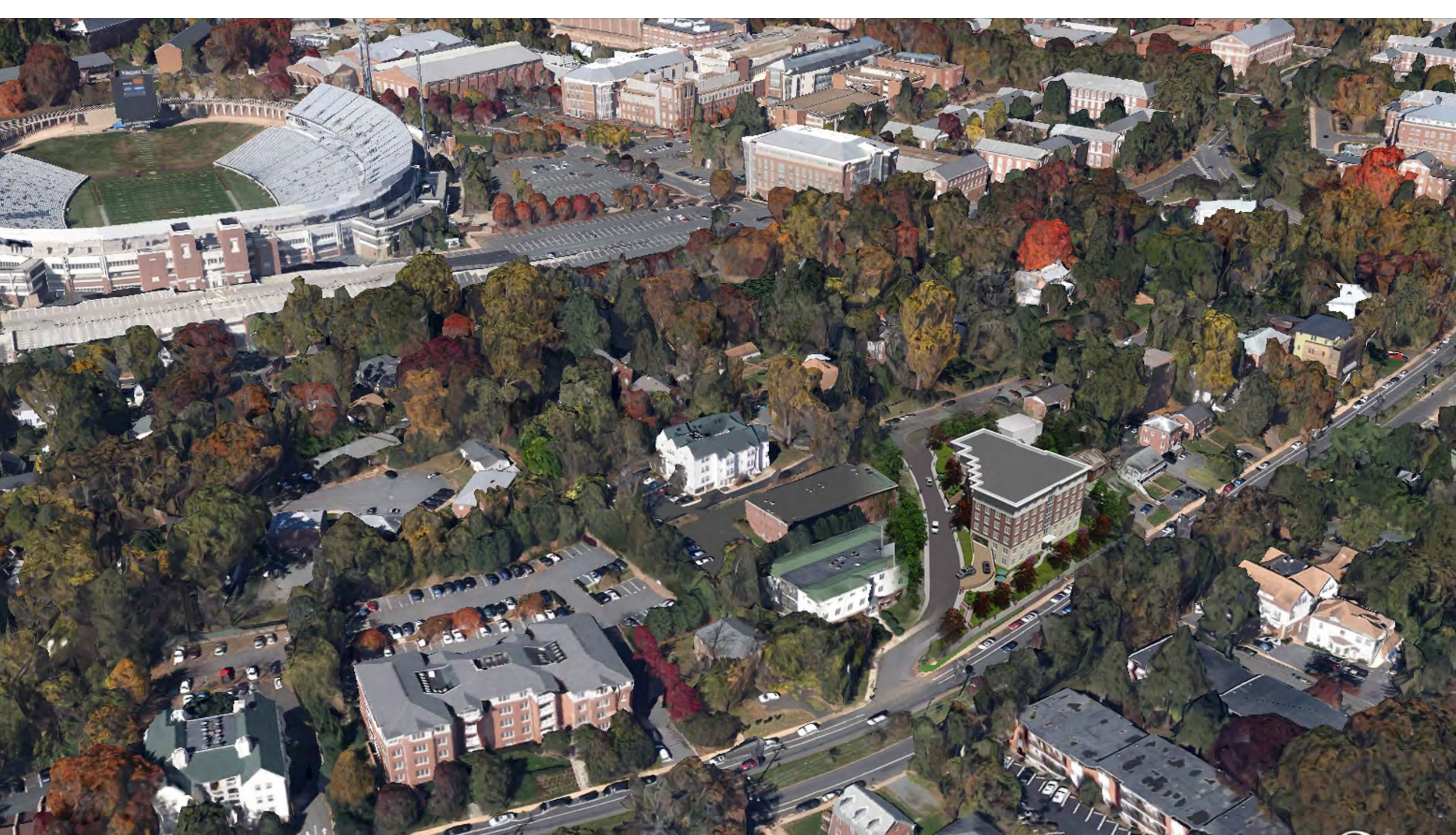
1725 JEFFERSON PARK AVENUE CHARLOTTESVILLE, VIRGINIA BIRDS EYE VIEW FROM SOUTH WEST
