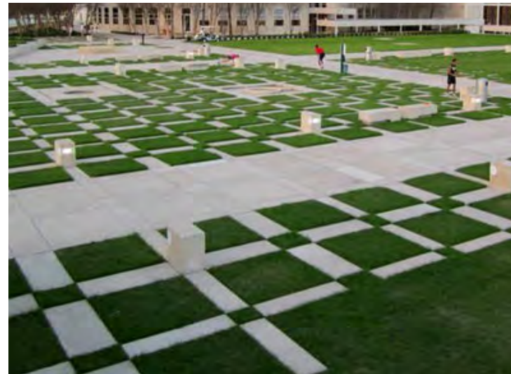
Paving with Lawn Joints and Panels
