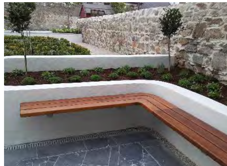
Cantilevered Wood Bench
