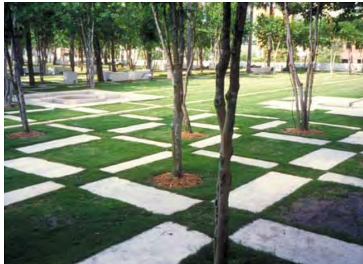
Paving with Lawn Joints and Panels
