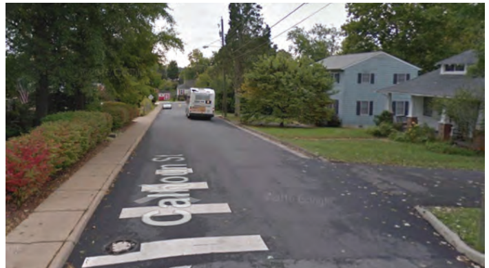
Calhoun Street between Locust and St. Clair – 30’ with parking allowed on both sides. Some driveways and a 4’-5’ sidewalk on the north side of the street.
