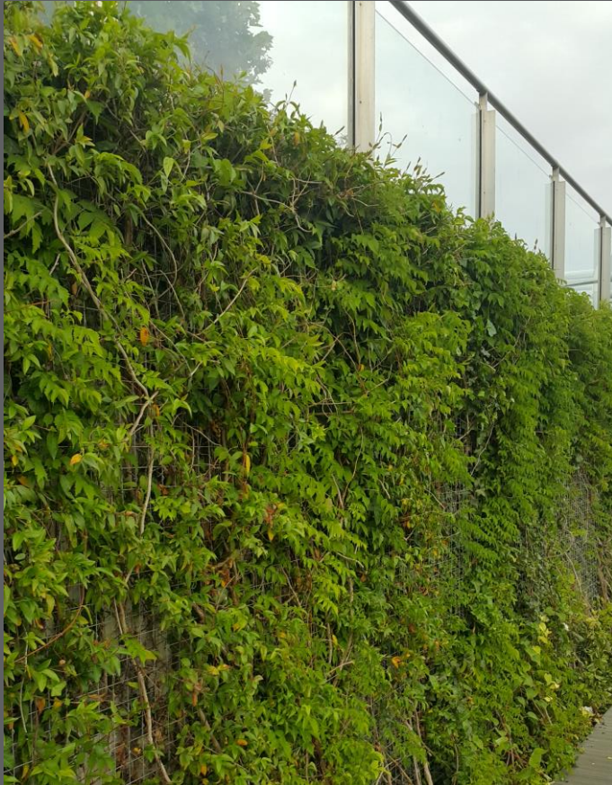
Trellis Panel on Masonry Wall
