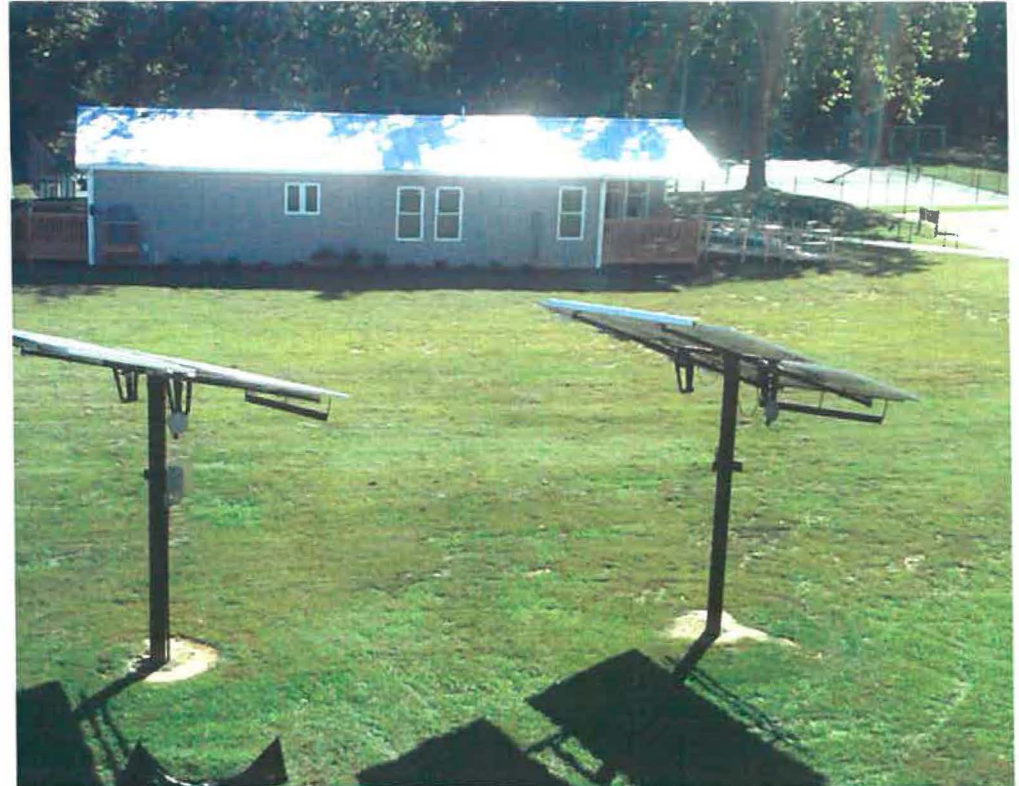
Two pole-mounted solar energy systems are installed at Charlottesville High School
