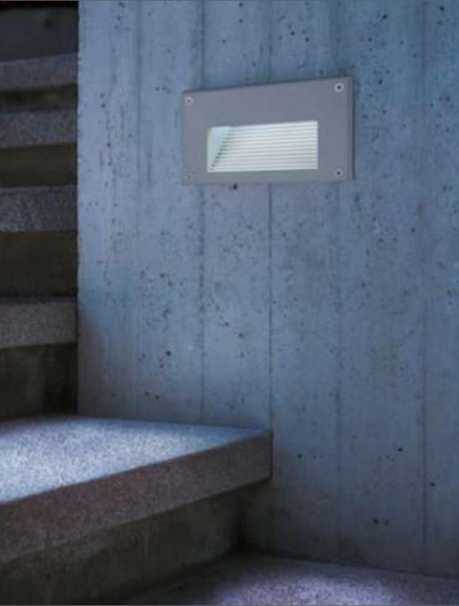
Recessed Wall Fixture at Parapet
