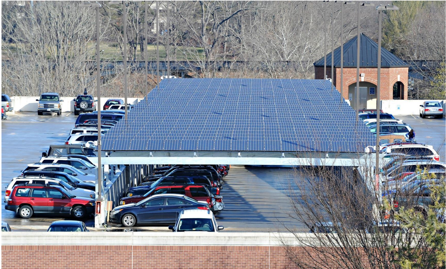
Parking Garage Canopies
