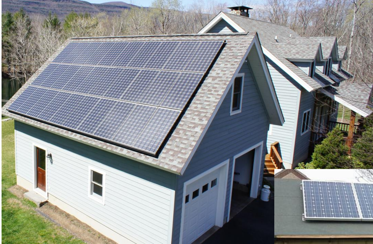
Mounted on garages and sheds
