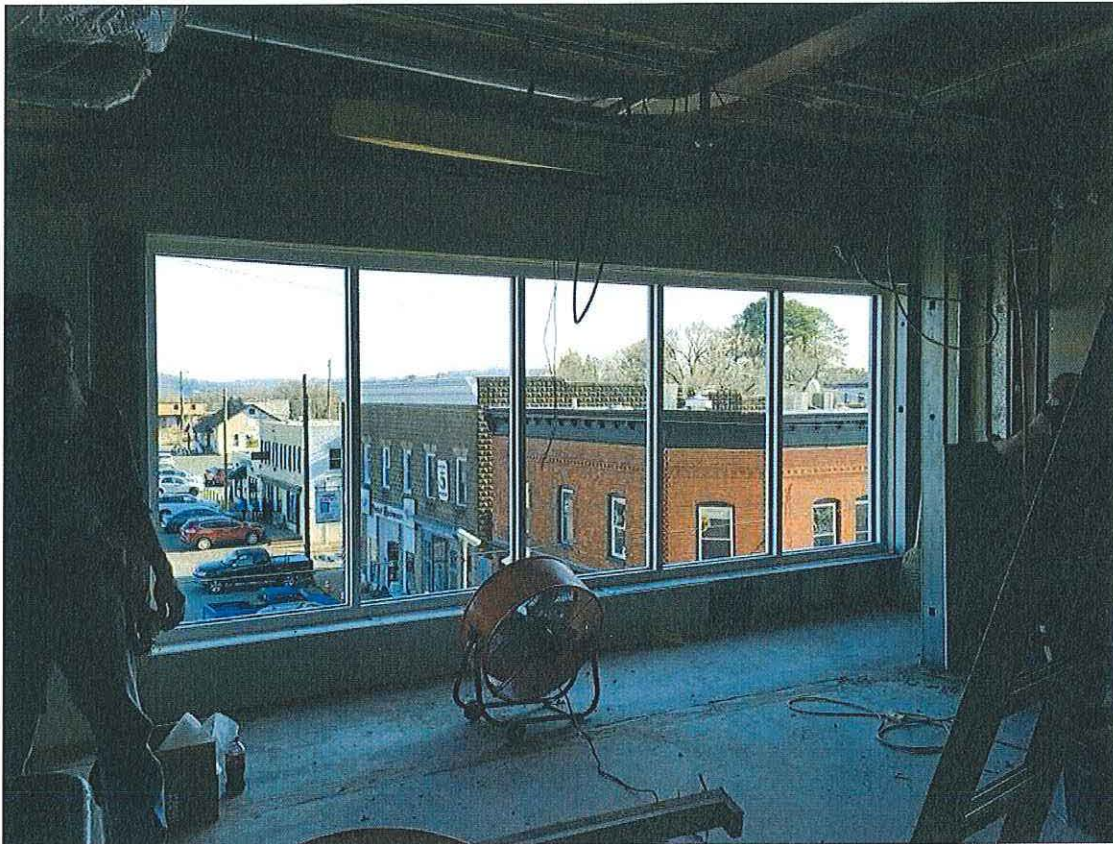
New windows now enclose the balcony area in the Common Area.
