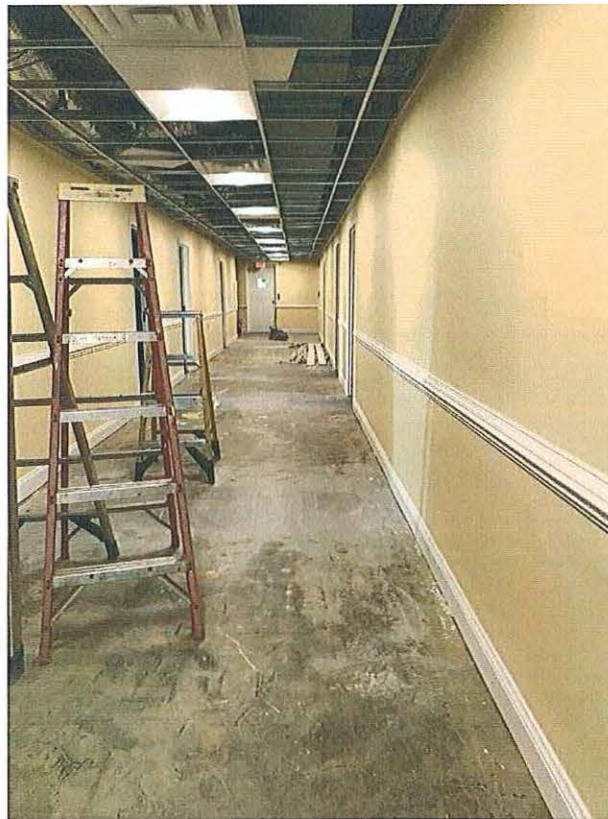
New floors are going in next!
