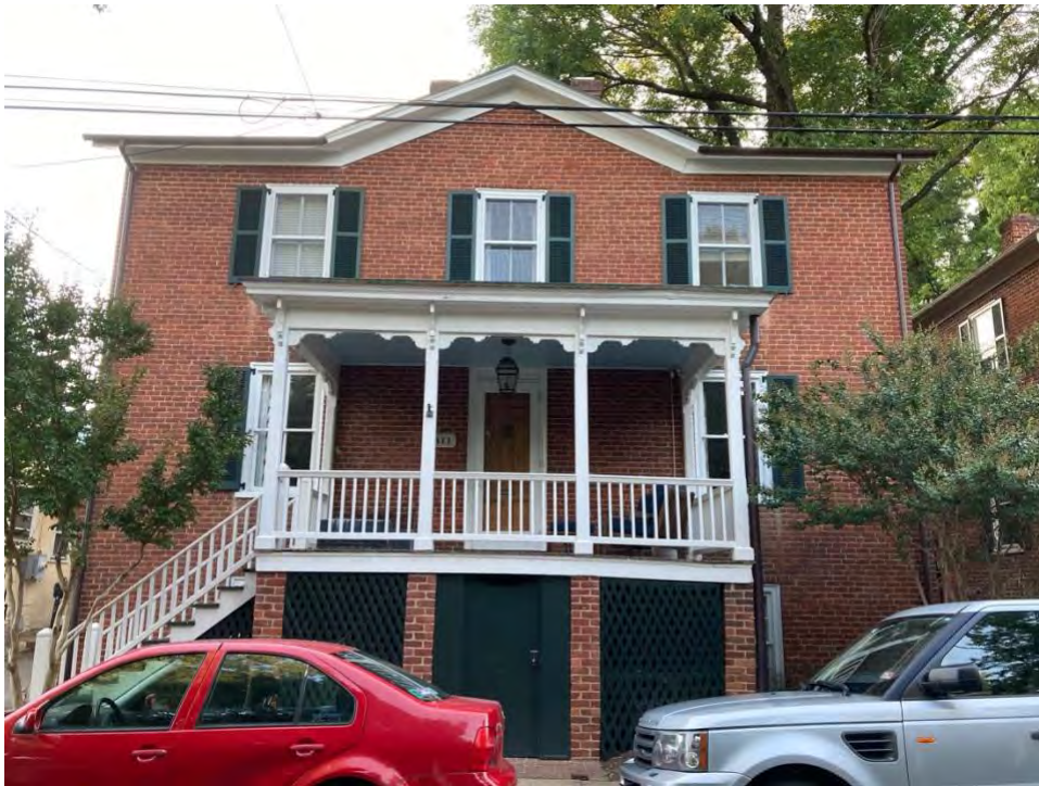
Figure 2: East elevation of 411 North 1 st Street.
