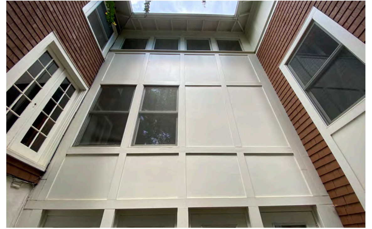
3. 1996 ADDITION - SOUTH ELEVATION - DETAIL OF WOOD PANELING
