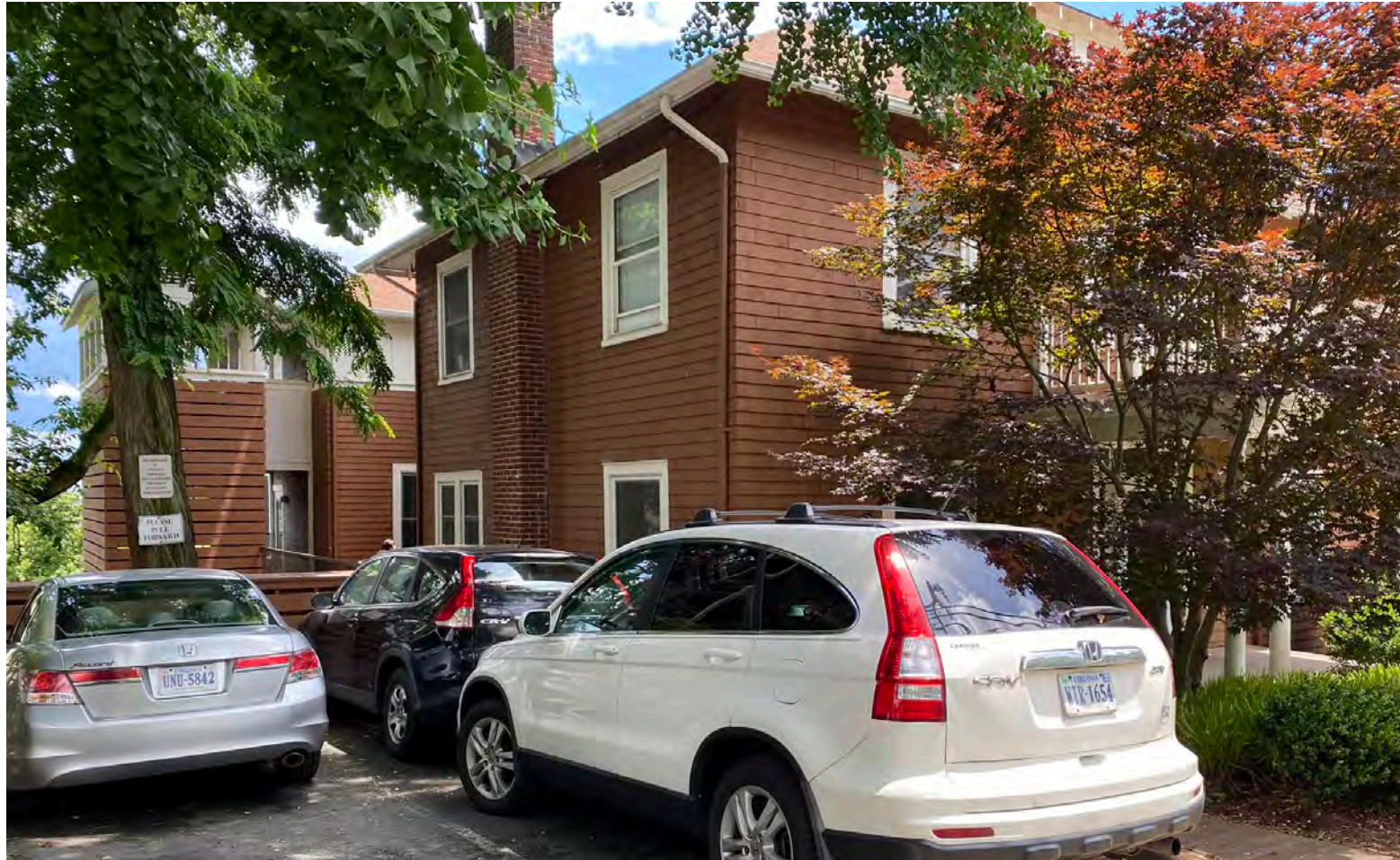
Existing view from Chancellor Street sidewalk
