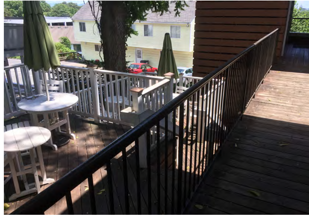
2. NORTH WOOD DECKS
