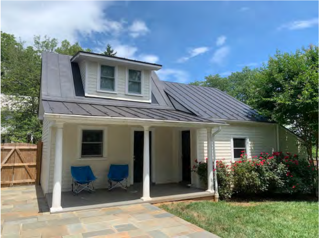
Another view of the garage/guesthouse, taken from behind the primary structure.
