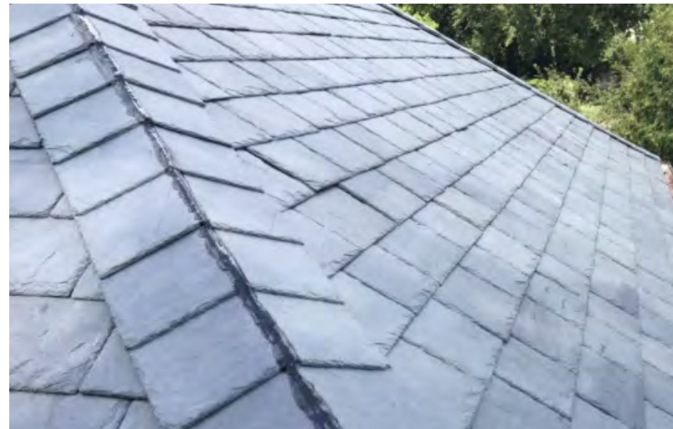
HIP DETAIL (BELLAFORTE SLATE)
