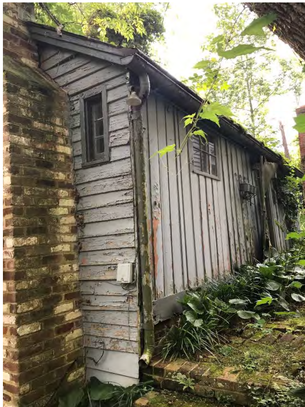
Cottage view from driveway
