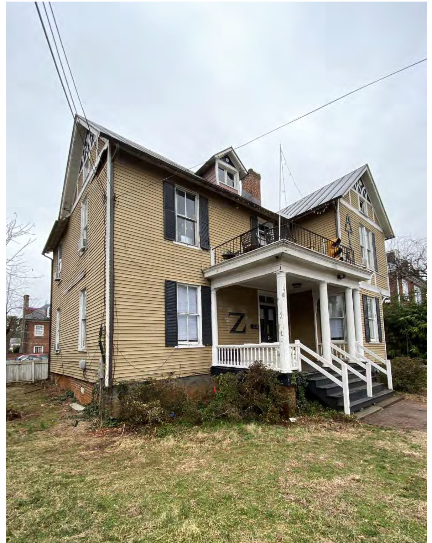
Existing Exterior S/E FRONT OF HOUSE
