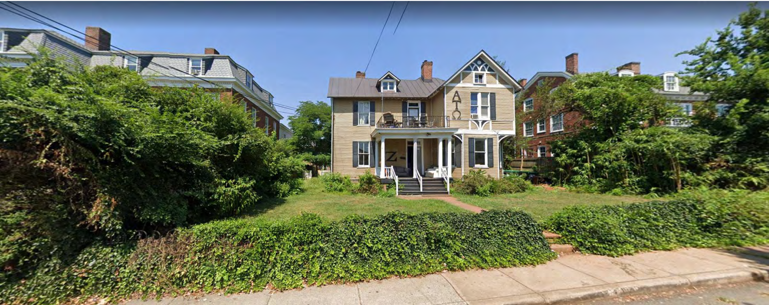
Existing Exterior Context VIEW FROM CHANCELLOR ST
