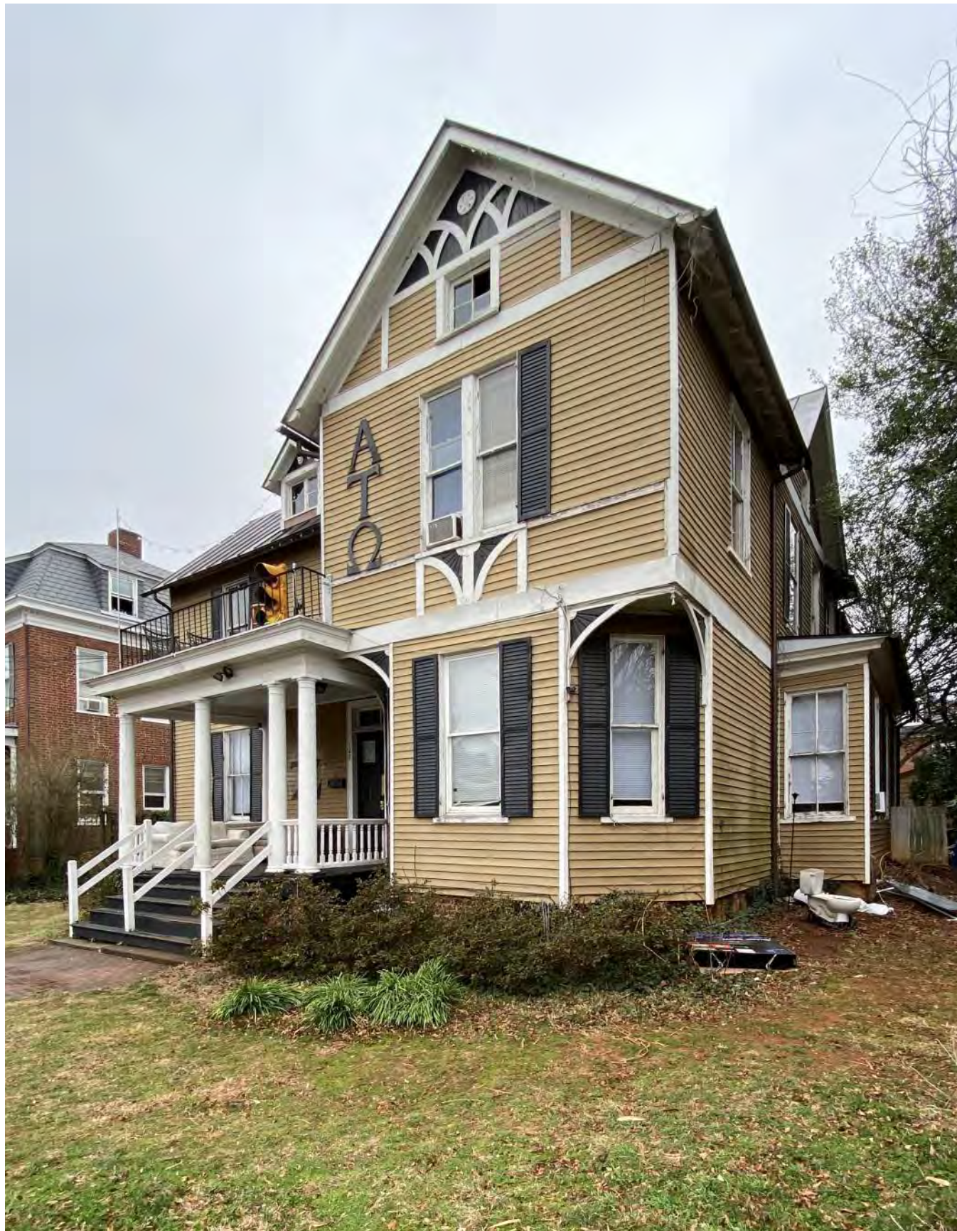
Existing Exterior N/E FRONT OF HOUSE
