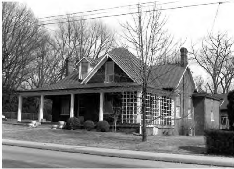
734 LOCUST AVE: PHOTOGRAPH FROM THE 1950s (SOURCE HISTORIC SURVEY)
