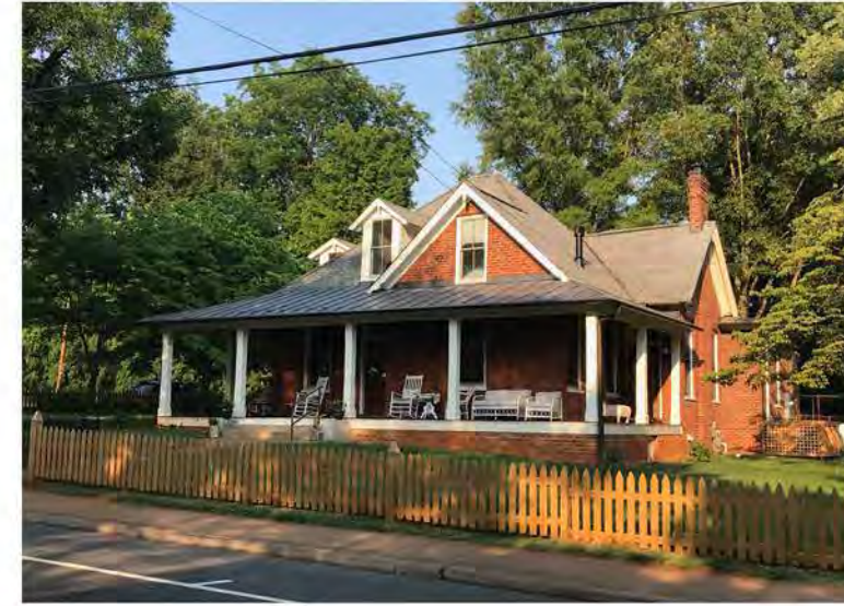
FRONT POST RENOVATION, SUMMER 2021 (SOURCE: G+G)
