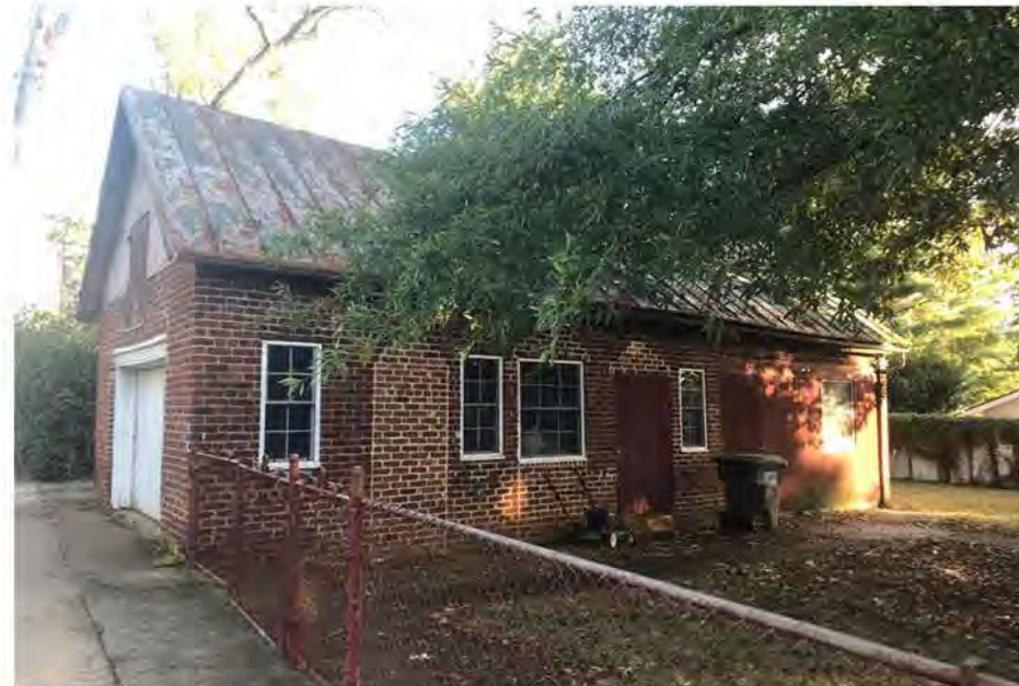
BACKYARD & HAZEL ST FACADE
