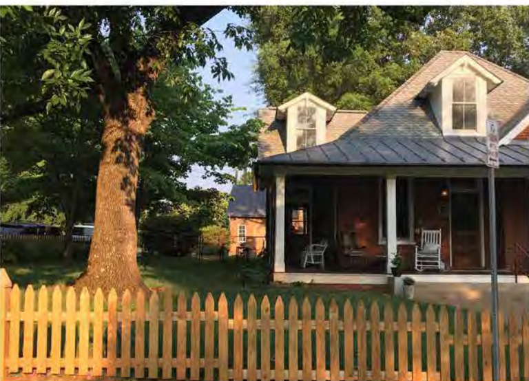
VIEW FROM LOCUST AVE TO CARRIAGE HOUSE (SOURCE G+G)
