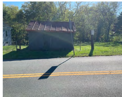
1800 Shed at street (further west)
