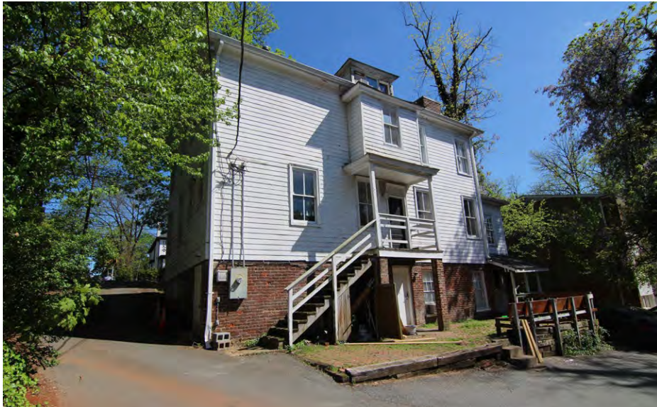
Parking area facing South-East
