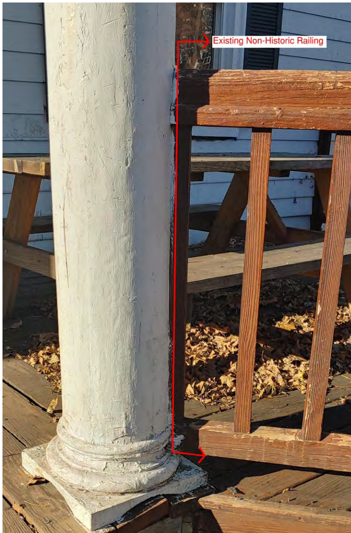
Existing Historic Column Base
