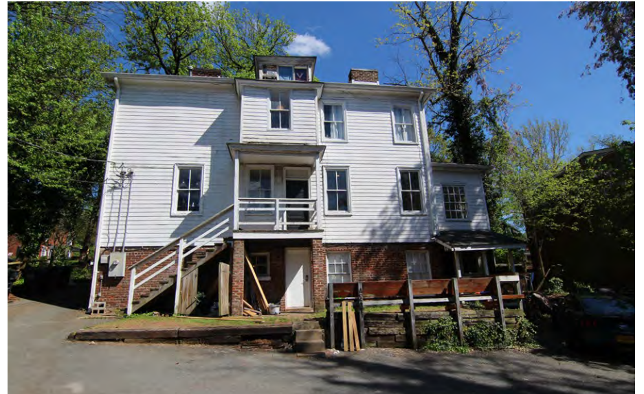
Parking area facing East
