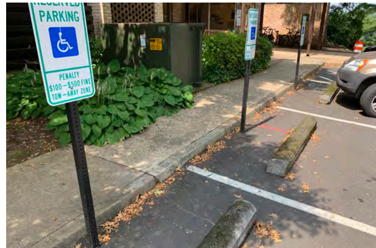
ACCESSIBLE PARKING SPACE SIGNS SUBJECT TO DAMAGE FROM VEHICLES
