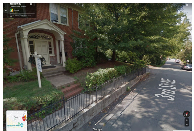
6. Brick two story, steps from sidewalk and at porch
