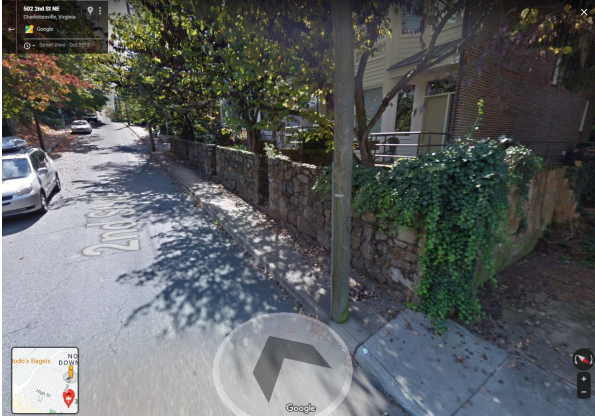
37. Tall stone retaining wall at sidewalk
