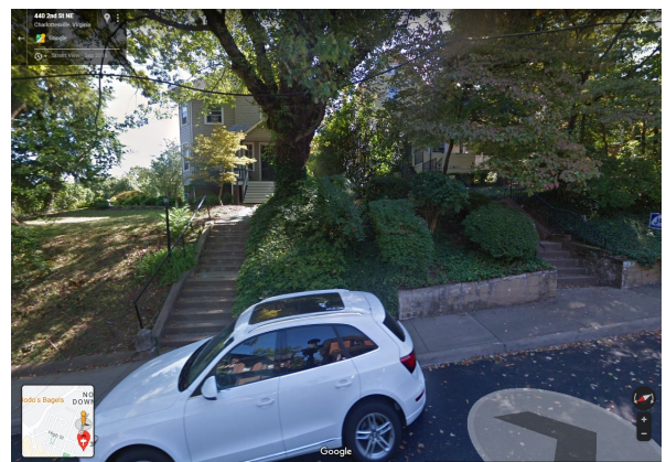
34. Concrete steps up and steps up to front porch (approx. 20 steps)
