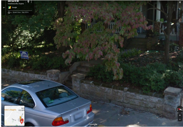
31. Stone retaining wall against sidewalk with steps up, and then more steps up to porch
