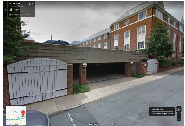
2. Garage and fence gates against road (Queen Charlotte)
