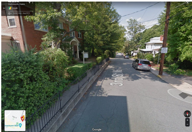
5. Wrought iron detailing against sidewalk w foundation plantings beyond
