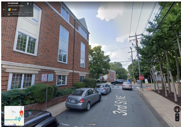
3. Foundation plantings between sidewalk and building (Queen Charlotte)
