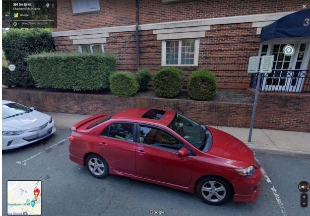
1. Brick retaining walls against sidewalk to reduce height of foundation (Queen Charlotte)
