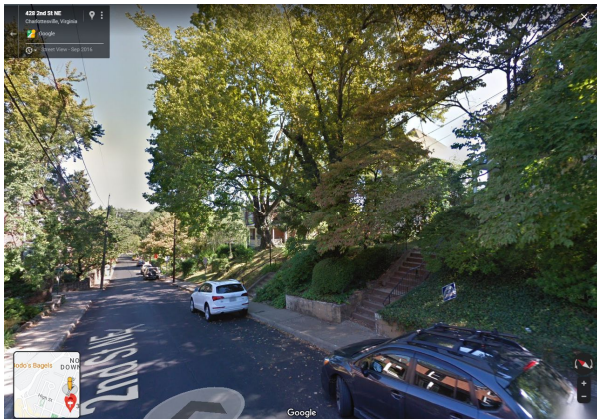
33. Concrete retaining wall with multitude of steps up
