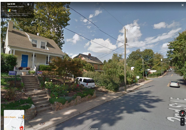
41. Stone retaining wall against sidewalk with steps up to front porch (approx. 20 steps); and driveway to right of house
